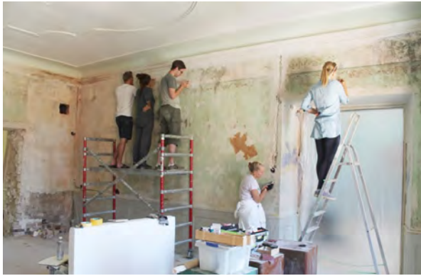
Photos depicting the process of revealing the green paint layer. Photos: Anna Holmberg
