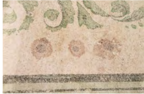
Recently placed plaster in 3 damaged spots on the south wall. Photo: Viktor Källgren
