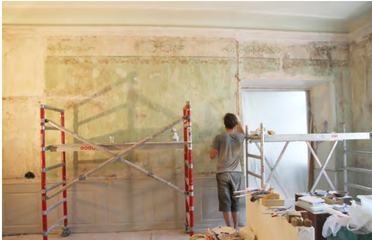
Work with filling holes with plaster continued. Photo: Rebecca Vemdal
