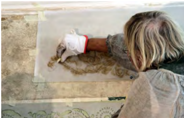
Heli is using a sachet with pigment to attach it to the wall using the pinned through stencil. Photo: Viktor Källgren
