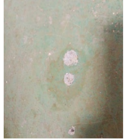
Air pumping the dirt away from the holes. Pictures of holes on the W-wall painting and holes filled up with plaster. Photos: Josefine Israelsson
