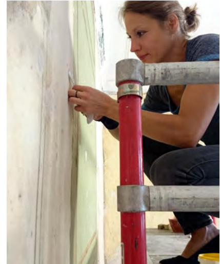
Filling of small holes in room N16. Photo: Vikoria Arvidsson
