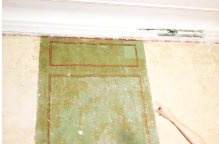
Wallpaper glue residues test cleaning. Photo: Anna Holmberg
