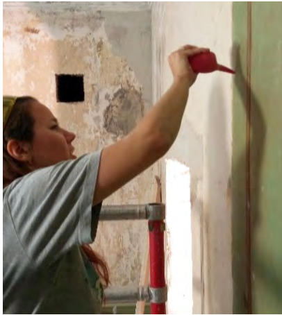
Air pumping the dirt away from the holes. Pictures of holes on the W-wall painting and holes filled up with plaster. Photos: Josefine Israelsson
