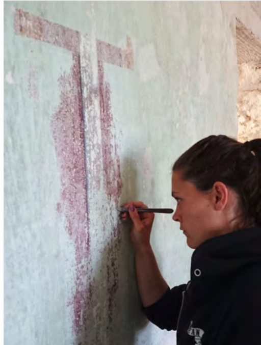
Right: Student scraping paint to reveal flower ornaments on the east wall.
