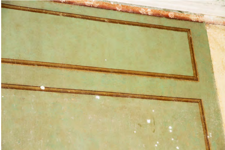
Dried plastered holes ready for retouching with paint. Photo: Rebecca Vemdal
