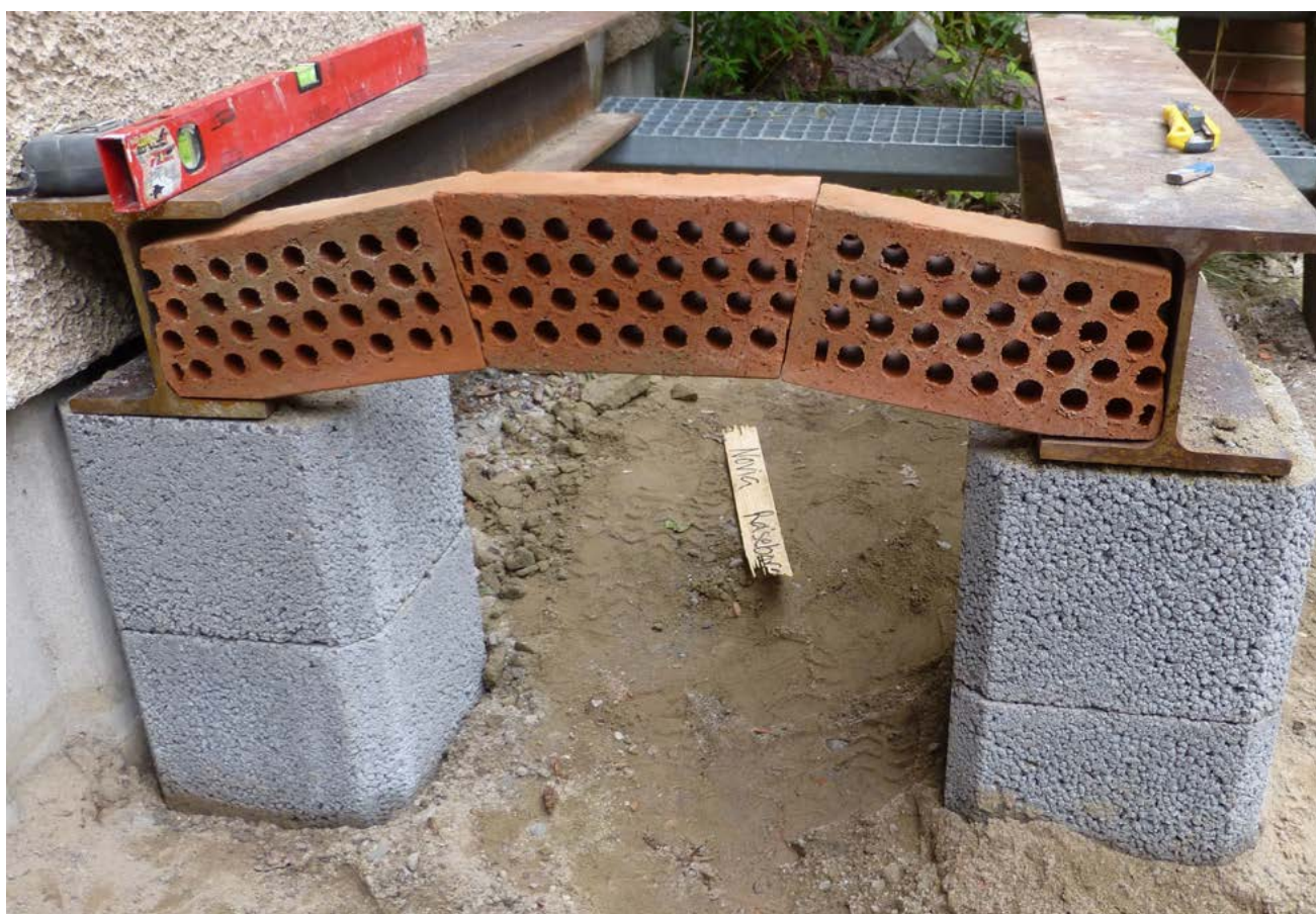
FIGURE 2.21. The shape of each brick was carefully measured and cut to make a flat vault. Photograph by Kirsti Horn.
