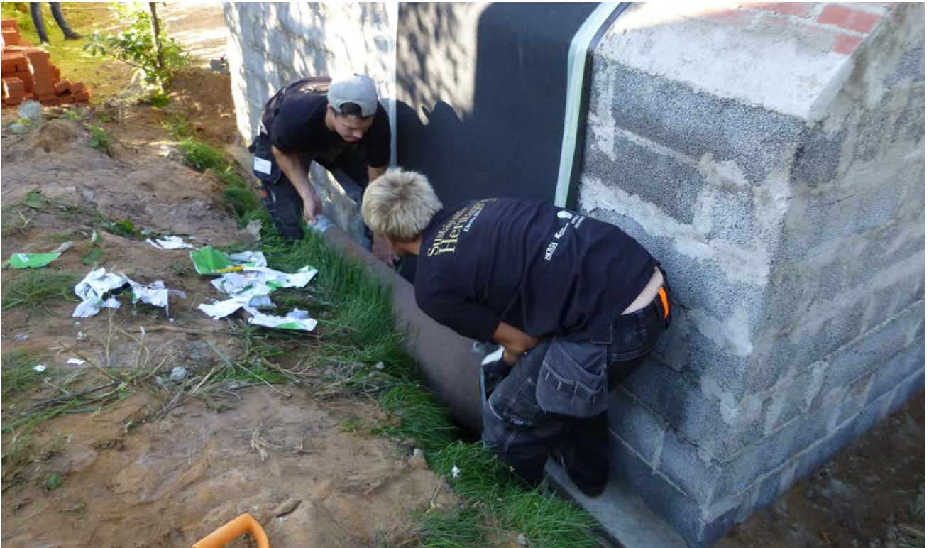
FIGURE 2.25. The felt is being measured long enough to protect vault, walls and the top of the plinth from rainwater. Photograph by Kirsti Horn.
