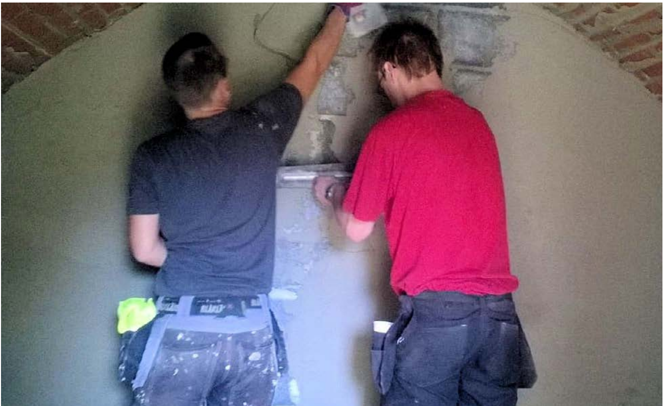
FIGURE 3.2. Plastering a wall takes a lot of practise. These students obviously knew the trade. Photograph by Kirsti Horn.
