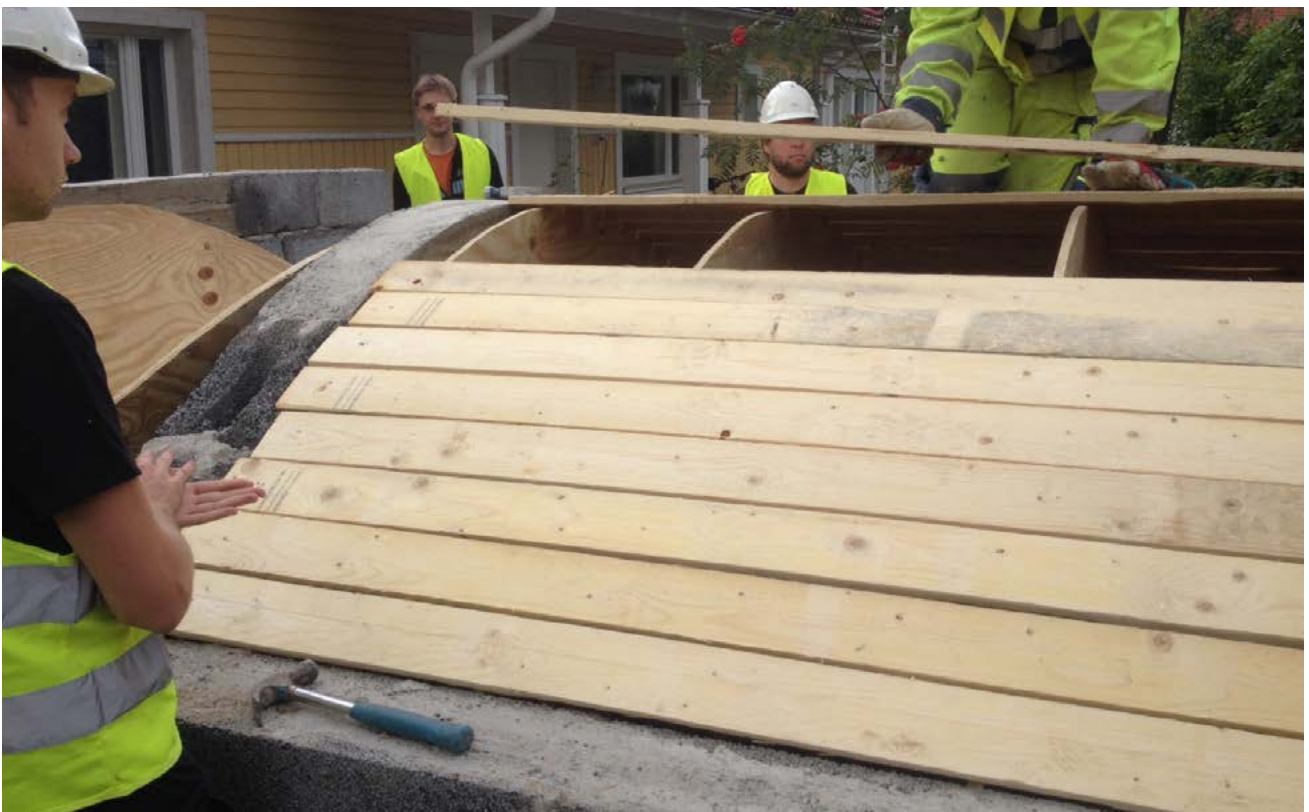
FIGURE 2.14. The centering for the storage room vault is completed by boards nailed onto the plywood sheets. Photograph by Sanna Svensson.
