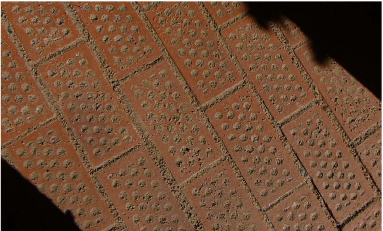
FIGURE 3.7. The finished floor is both functional and beautiful. Photograph by Kirsti Horn.
