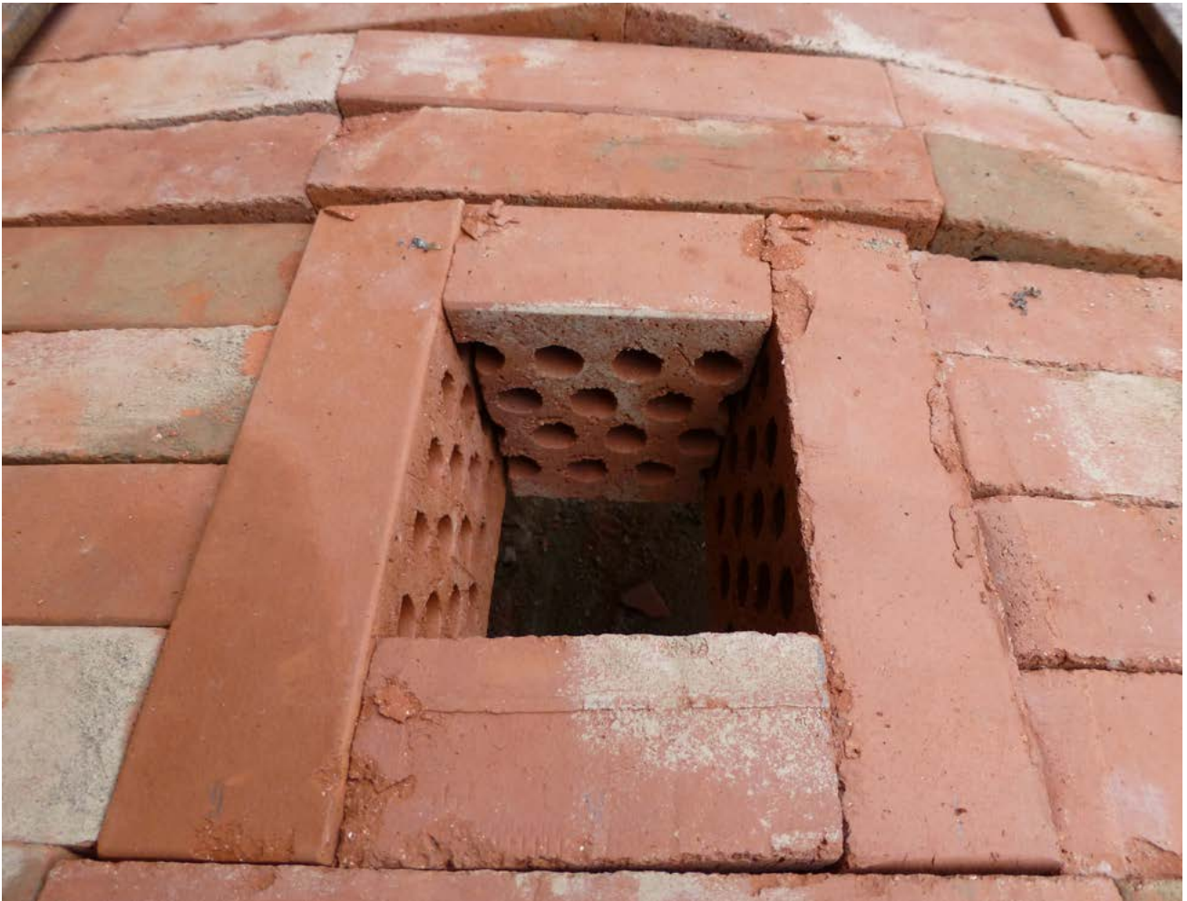
FIGURE 2.24. Note how the two back rows are made with waste pieces from the bricks of the front rows at the ends. Alternating the two types would give a stretcher bond. Photograph by Kirsti Horn.
