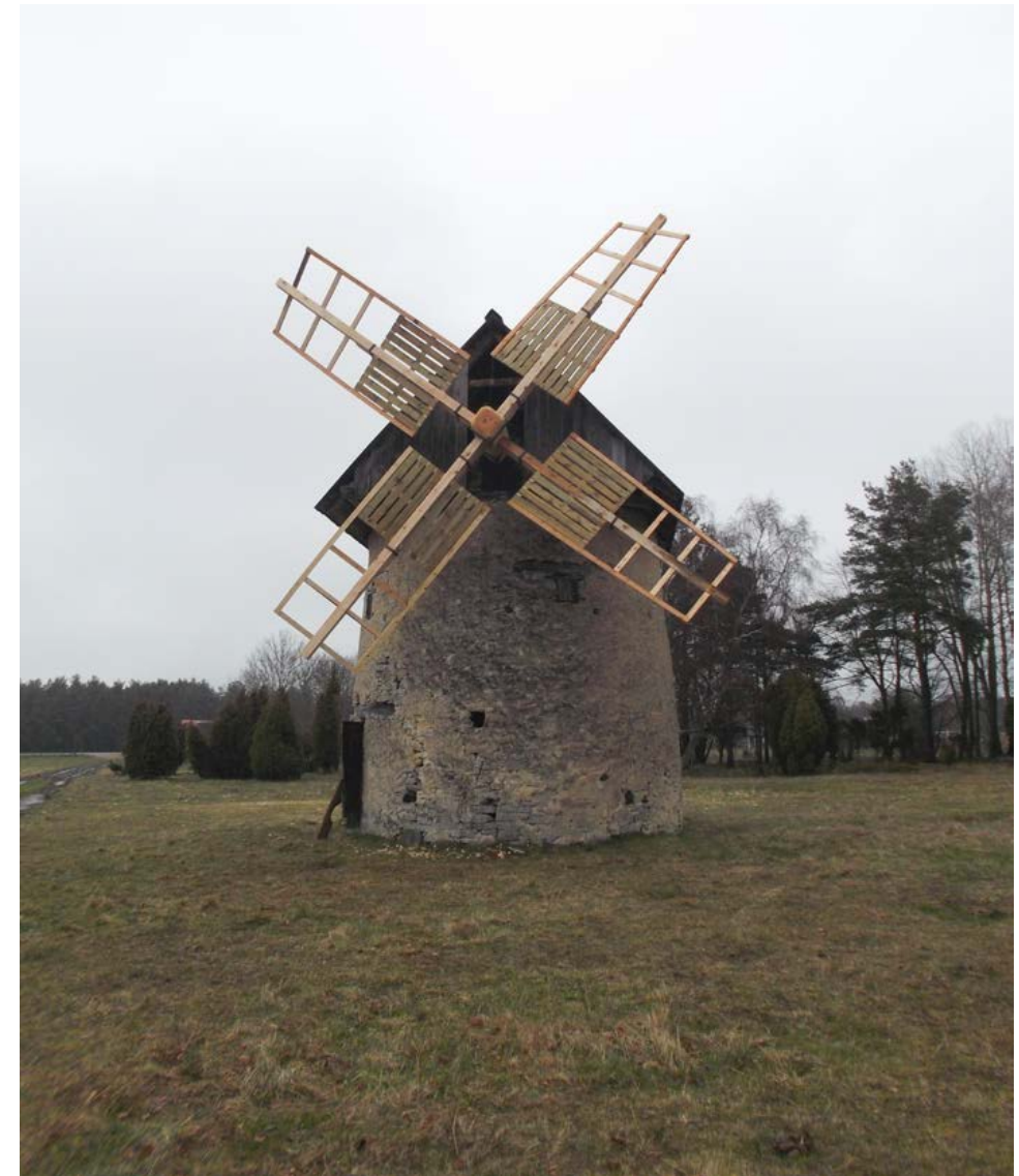
Figure 1.24. After three days of intensive work the windmill at Sieger farm was more complete than before. The performed repairs were the first steps in a restoration process where a lot more would have to be done before cereals could be ground. Even if only mock sails were built at least the wind shaft will last another century or two! Photograph by Kenneth Eriksson.
