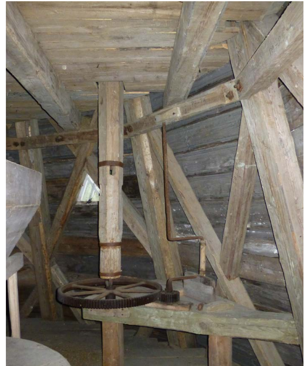
Figure 7.2. View of first floor or stone floor behind the two pairs of stones. The hand winding to turn the cap was done from here with the help of the iron crank which turned an upright wooden shaft next to it via an iron pinion and wheel. Oripää mill, Seurasaari, Helsinki. Photograph by Kirsti Horn.
