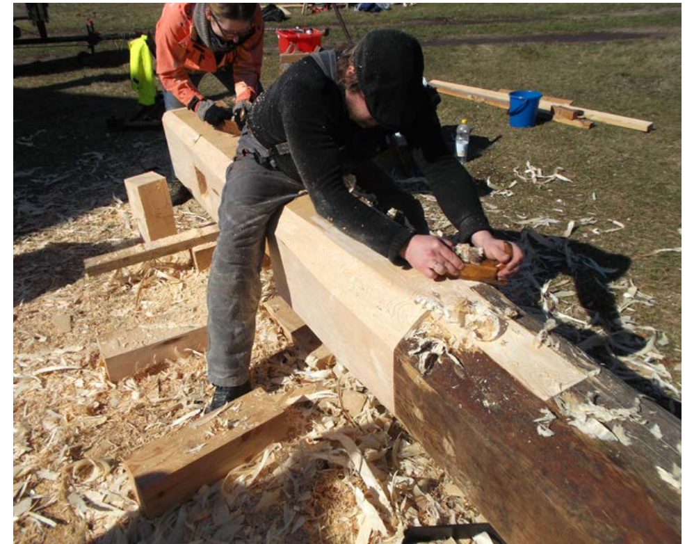
Figure 1.12. The surface of the new part of the wind shaft was planed smooth with hand tools. Photograph by Kenneth Eriksson.
