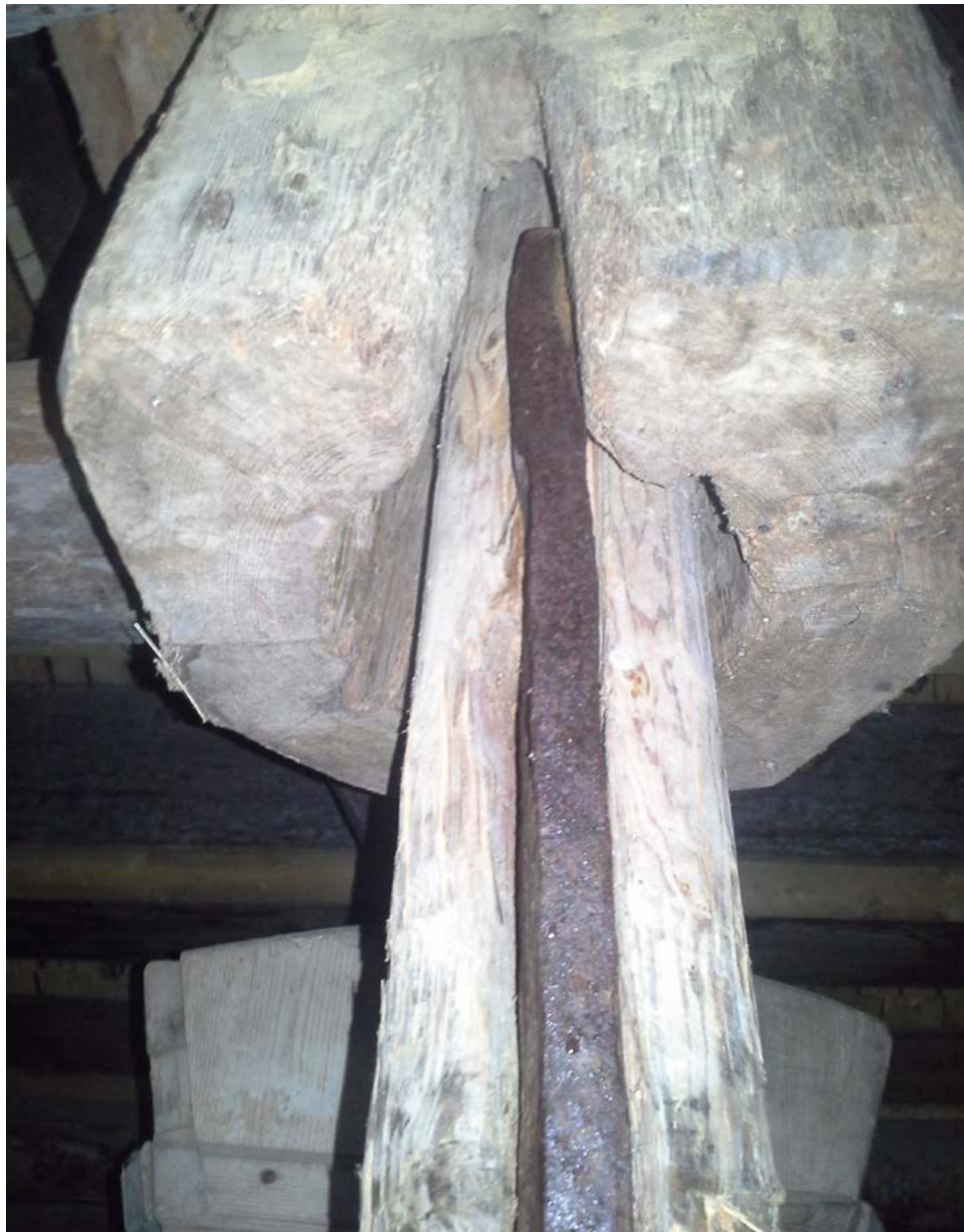
Figure 6.4. The upright hollow post inside which the upright shaft of iron is fitted enables the turning of the top while the lower part of the mill is immobile. Photograph by Gustaf Lindroos.
