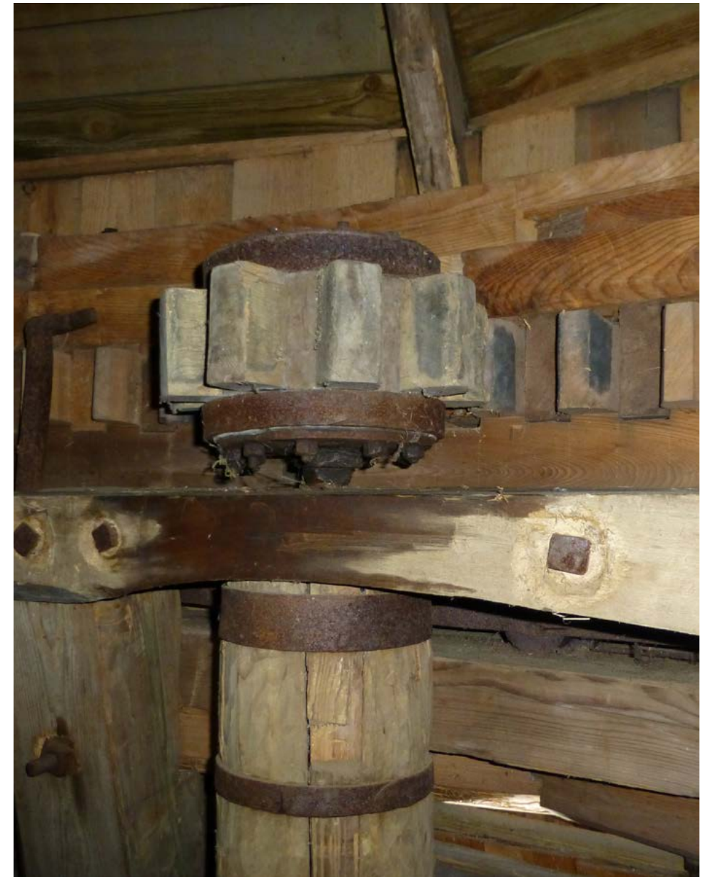
Figure 7.4. On third or top floor yet another pinion turned the cap which is fitted with cogs at the bottom edge. Oripää mill, Seurasaari, Helsinki. Photograph by Kirsti Horn.
