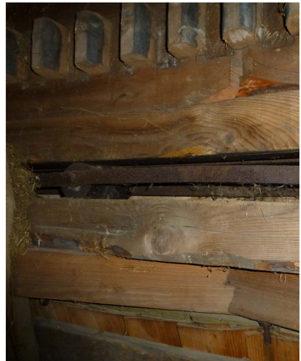
Figure 7.6. The curb between the body of the mill and the cap is fitted with small wheels. Today all the metal parts of the mill would need a thorough cleaning before the machinery or cap would move again. Oripää mill, Seurasaari, Helsinki. Photograph by Kirsti Horn.
