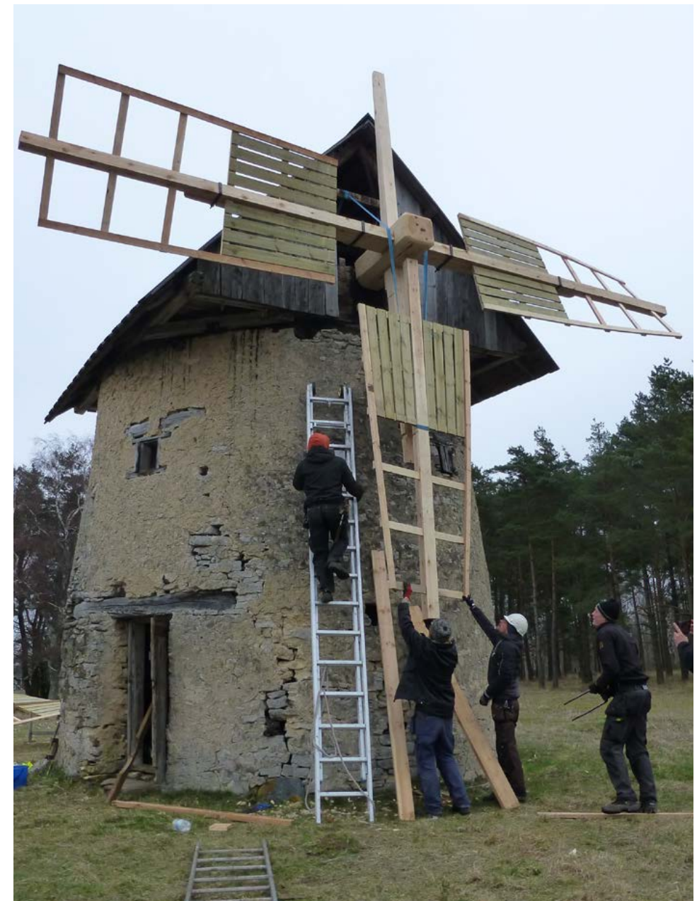
Figure 1.22. The sails were lifted one by one into position and attached with the original clamps. Photograph by Kirsti Horn.
