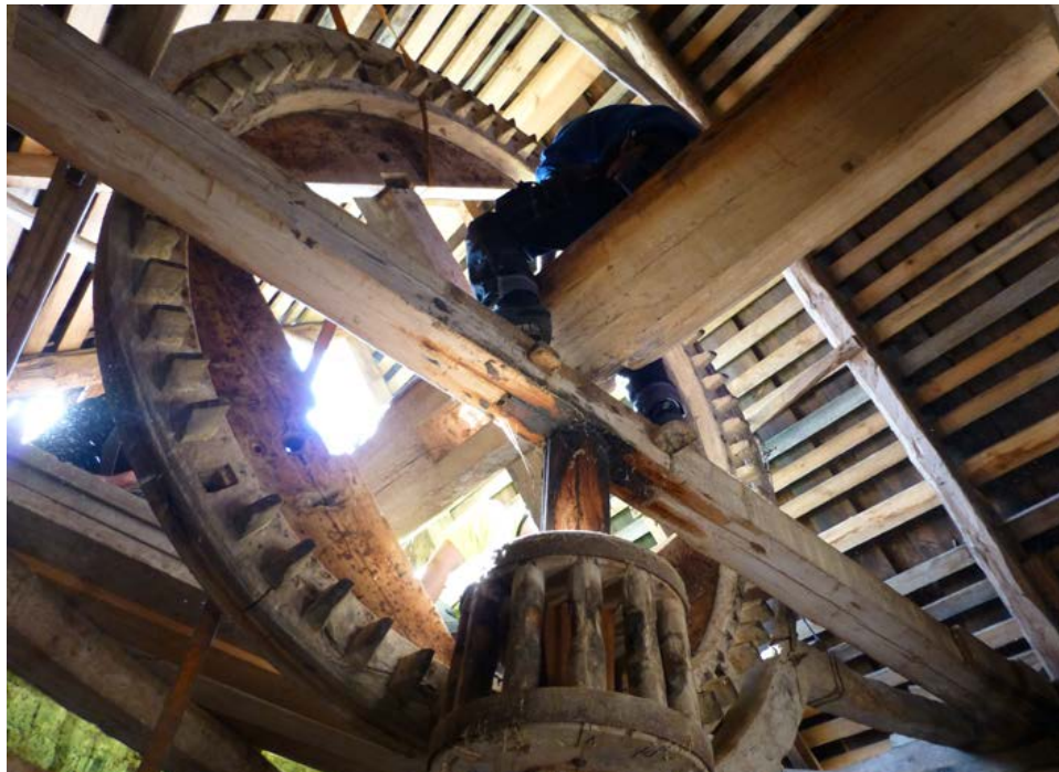
Figures 1.16 and 1.17. Views from front and back of the brake wheel being attached back to the wind shaft . Clouds of saw dust from woodworm appeared with every beat on the wood. Photographs by Kirsti Horn.
