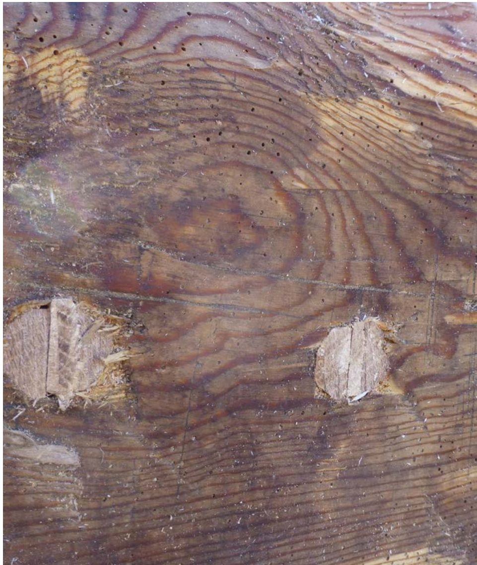
Figure 1.9. Two wooden pegs secure the joint between old and new parts. Wedges were forced in through their ends in order to tighten them. On the surface of the old wind shaft the bigger flight holes are made by Soft Wood Borers while the minute holes are made by Common Furniture Beetle. Photograph by Kirsti Horn.
