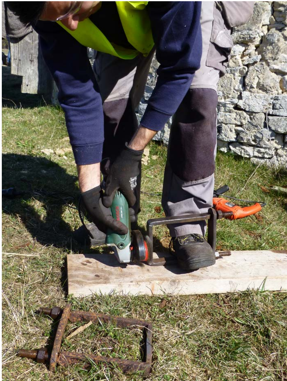
Figure 1.23. The original steel clamps were cleaned from rust before they were reused to attach the sails . Photograph by Kirsti Horn.
