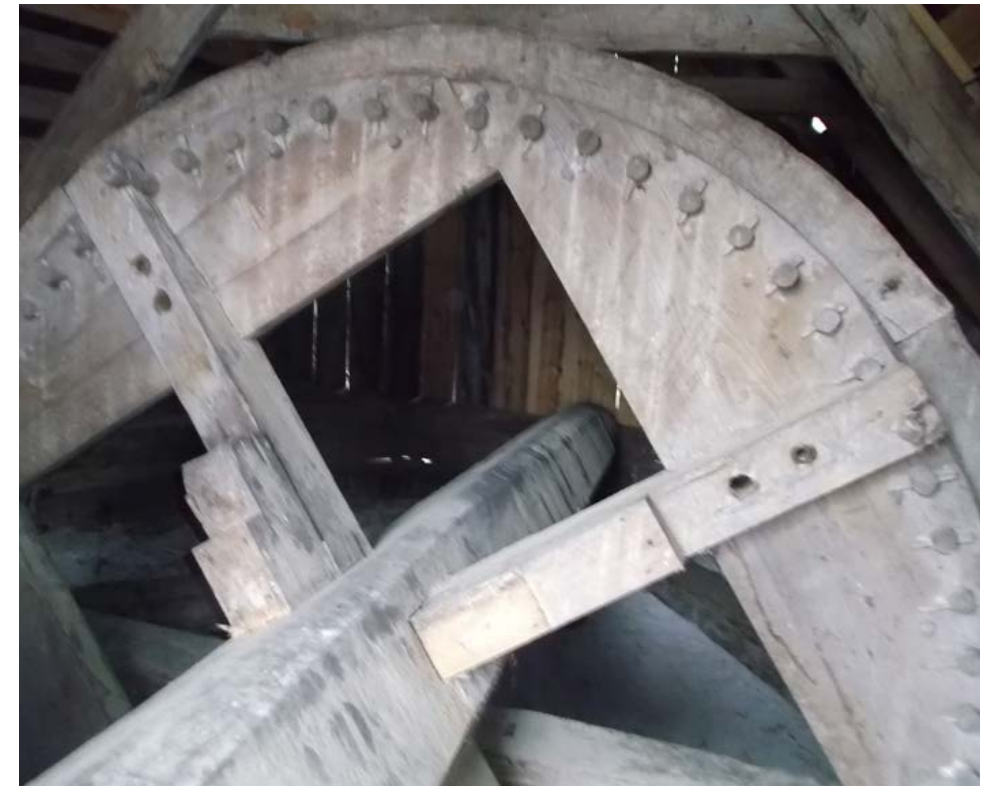
Figure 1.4. View through the brake wheel towards the rear end of the wind shaft . One wooden peg and one bolt have been removed from each spoke while the wedges are still in place. Photograph by Kenneth Eriksson.
