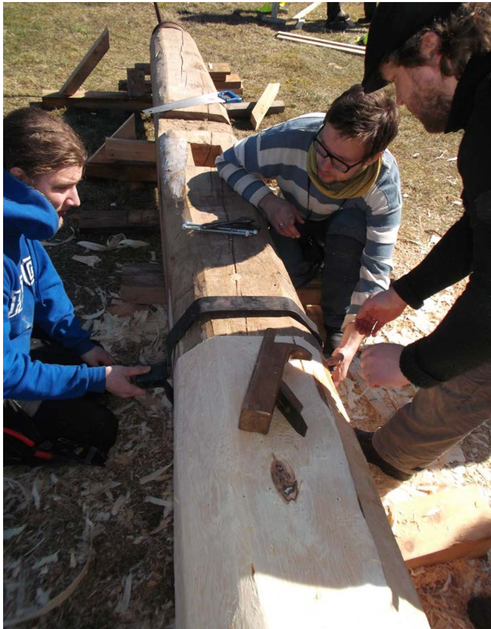
Figure 1.11. From left: John Friederich, Joosep Metslang and Dan Lukas are fitting the steel clamp around the joint between old and new sections of the wind shaft . Photograph by Kenneth Eriksson.
