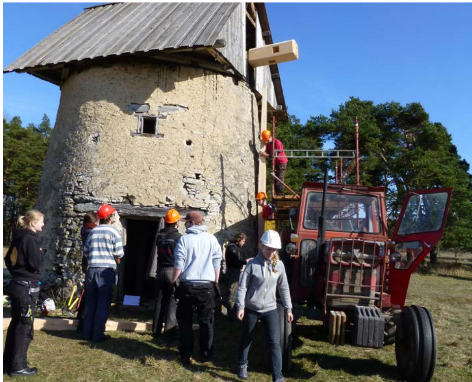
Figure 1.21. The heavy sail stocks were lifted and fitted through the eyes or sail stock mortices at the poll end of the wind shaft and secured with wooden wedges. Photograph by Kirsti Horn.
