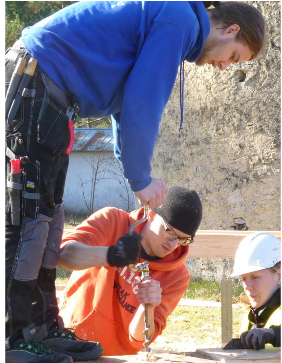
Figure 1.8. Two students are drilling holes for the pegs while the third is making sure the drill is kept straight. Photograph by Kirsti Horn.
