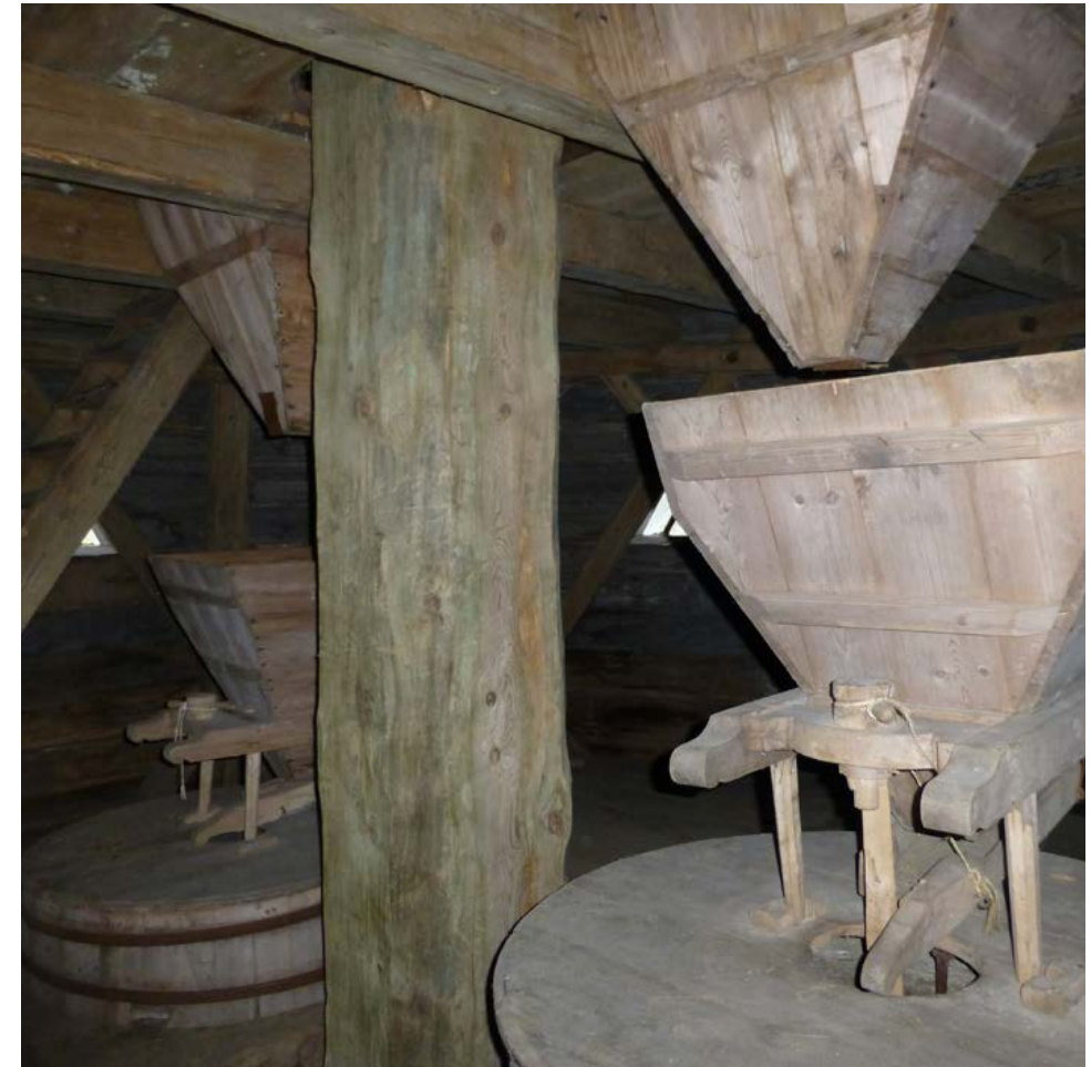
Figure 7.8. The two pairs of stones with their hoppers and troughs on either side of the sturdy upright shaft. Oripää mill, Seurasaari, Helsinki. Photograph by Kirsti Horn.
