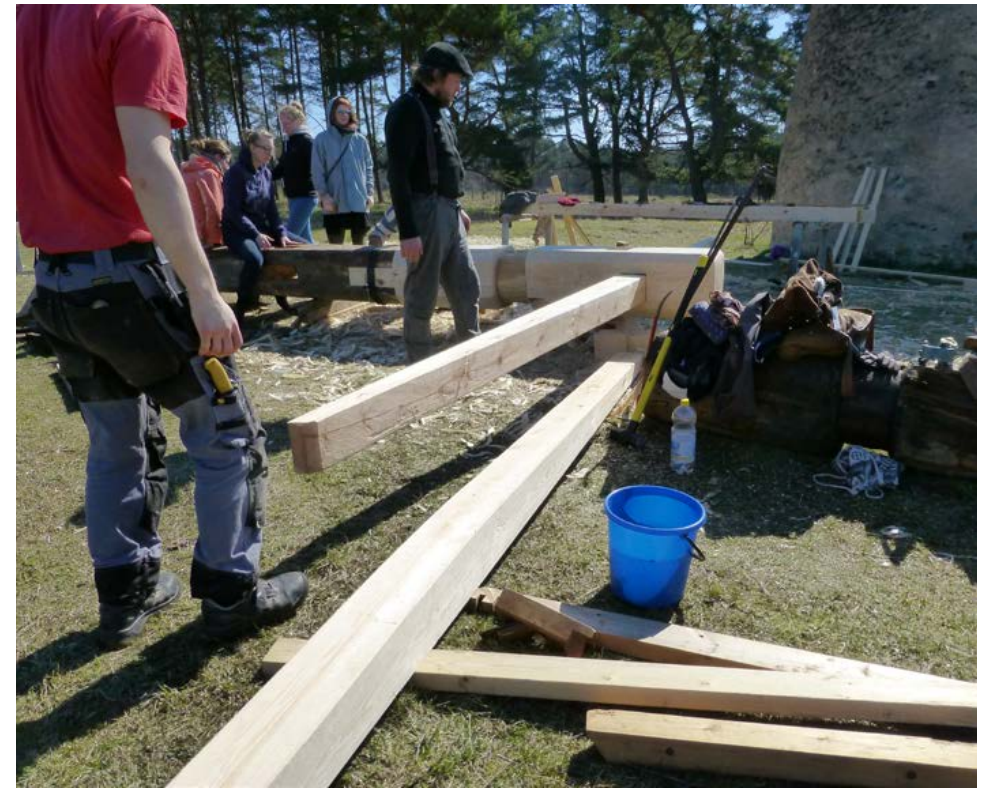
Figure 1.20. The two sail stocks were fitted into their holes at the end of the wind shaft before the shaft was lifted inside the mill. Photograph by Kirsti Horn.
