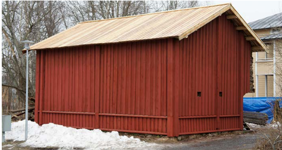
Figure 3.1. On the back of the loft the weatherboarding had to be patched. Vertical supports to the structure can be seen in the middle of the gable and at the far corner.
