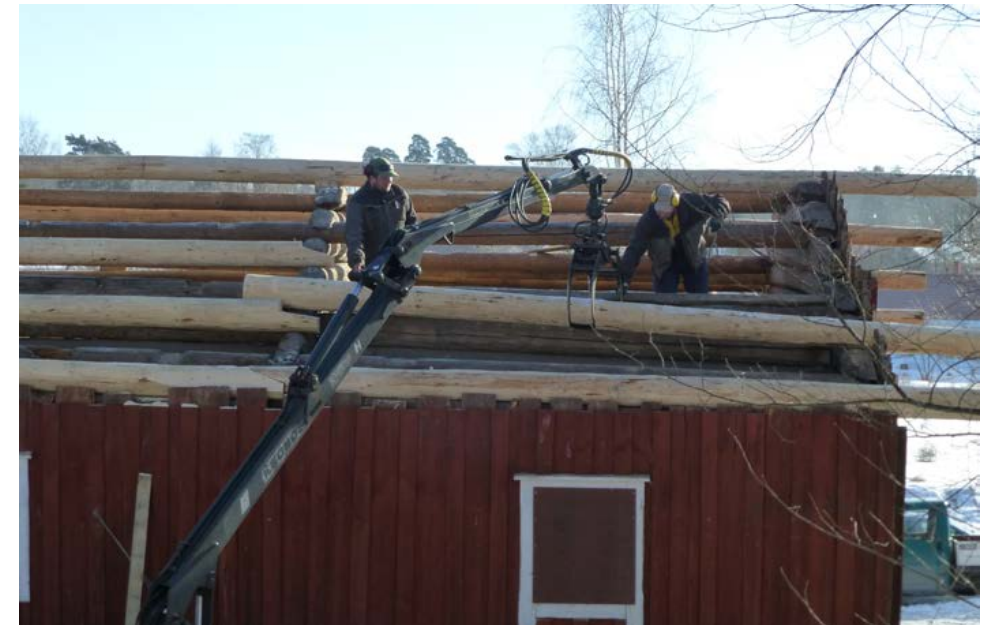
Figure P4. New purlins were installed by a construction company to carry the new roofing. Photograph by Kirsti Horn.
