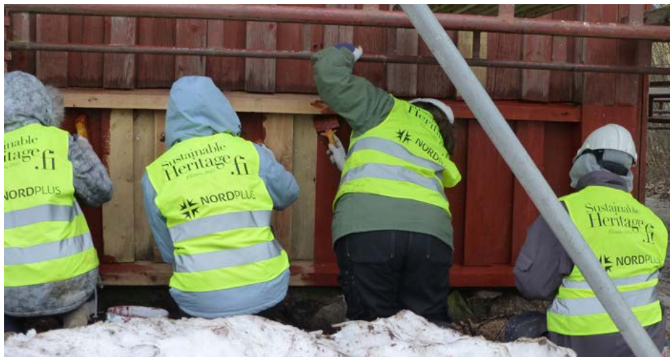
Figure 2.7. Applying red earth paint can be done even in bad weather. It is advisable to heat up the paint if the temperature is low. Photograph by Kirsti Horn.
