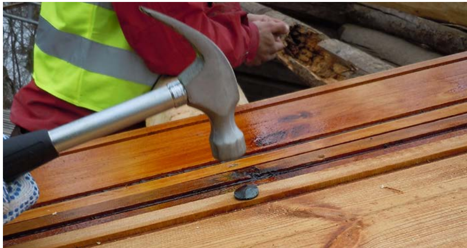
Figure 1.4. Banging the big nails into the purlins was hard work. Photograph by Siim Raie.
