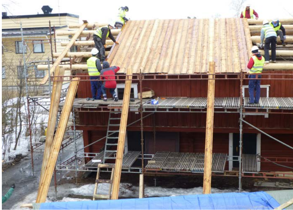
Figure 1.1. The security on the site was of obvious concern. Good scaffolding of steel bars and wooden platforms made it easy to move about on the roof. Helmets and safety vests are obligatory on a building site like this. Photograph by Kirsti Horn.
