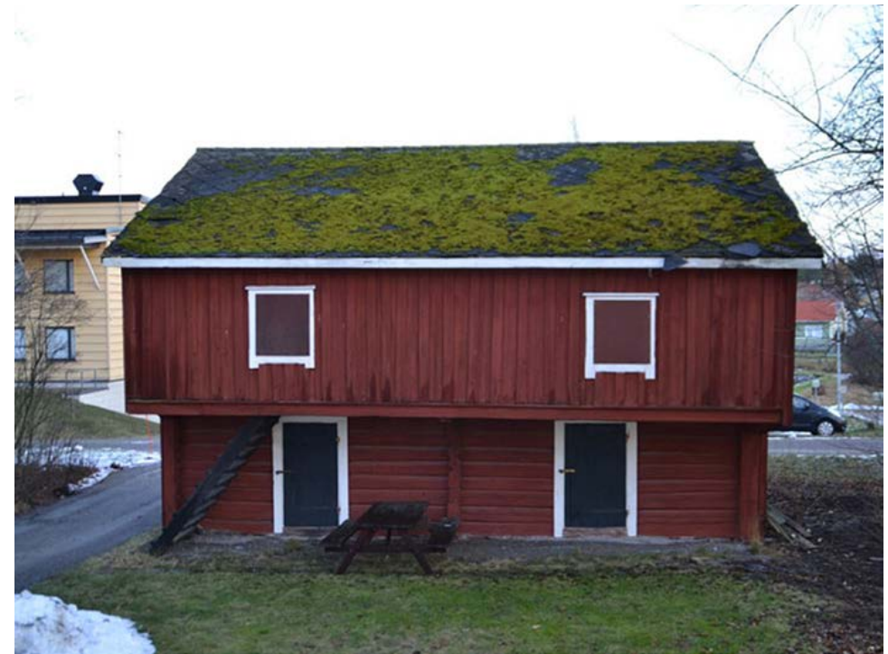
Figure P1. The broken roof of the historic loft was the starting point for the Wooden Roof project. Photograph by Niklas Nyman.
