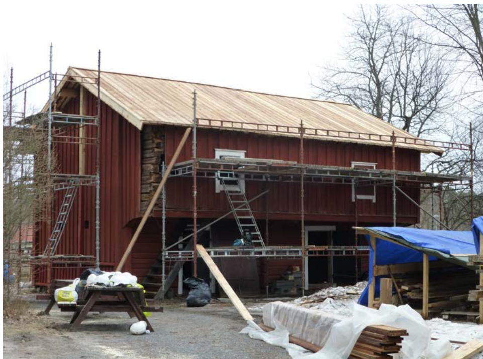
Figure 1.8. By lunch break on the fifth day the roof was complete while the paintwork on the façade still needed some finishing touches. The badly decayed front corner was secured at a later date. Photograph by Kirsti Horn.
