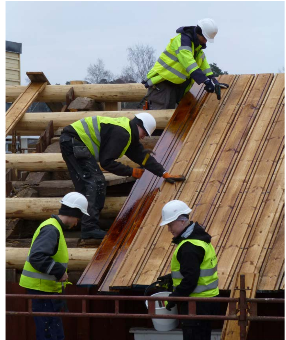
Figure 1.7. Drilling and nailing, drilling and nailing 650 times over.
