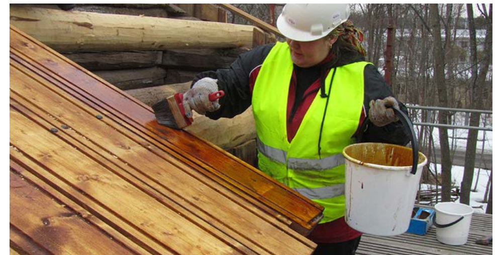
Figure 1.5. The bottom planks were tarred for the second time as the work went on. Photograph by Kaisa–Piia Pedajas.
