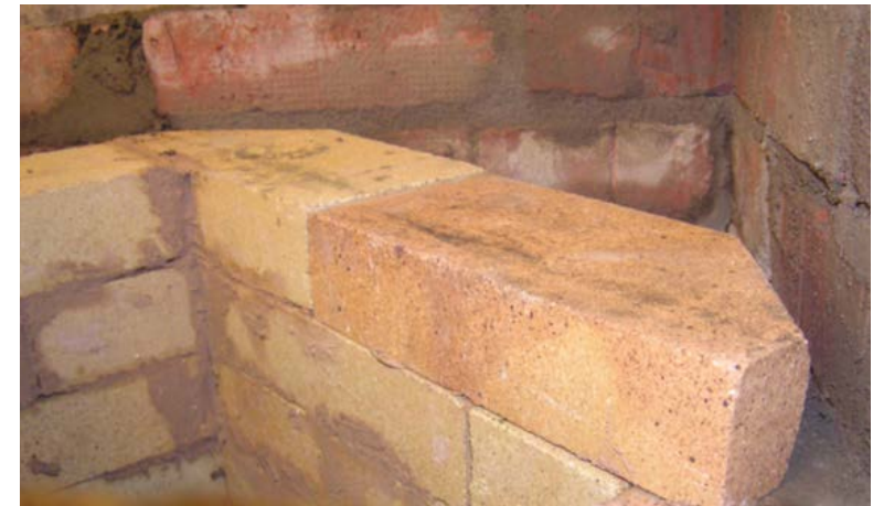
Figure 1.16. Fireproof bricks and mortar are used for the furnace. The bricks have to cover each cross-joint of the previous course.
