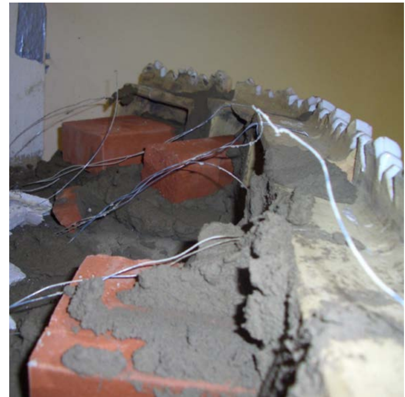
Figures 1.47–48. The chimney was repaired ( left ), before the crown tiles were finally inserted.
