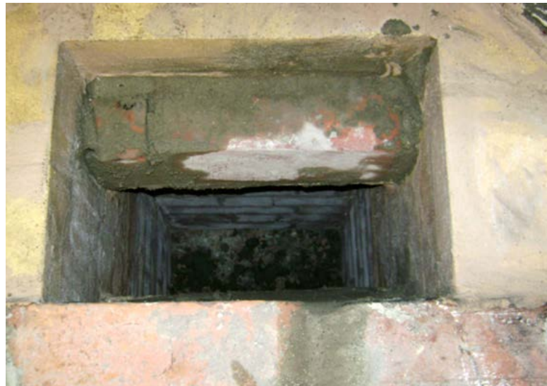
Figure 2.47. Behind tile row 8 the angle of the bottle neck of the middle flue has to be compensated in depth with approximately 50 mm of brick.
