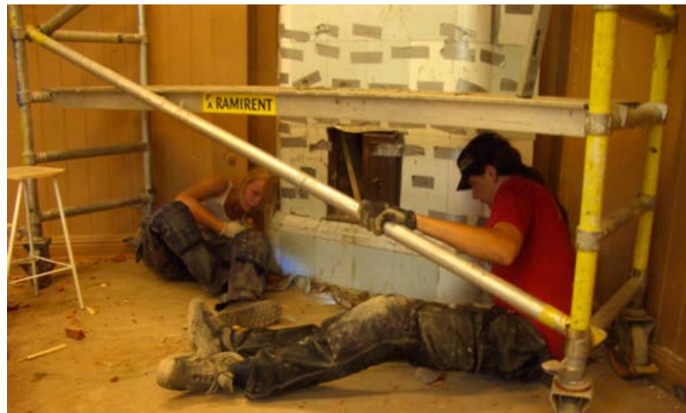
Figure 2.56. It is important to clean the bottom of the smoke flues from mortar droppings before the mortar sets!
