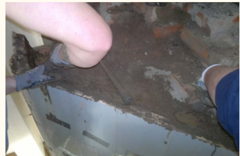
Figures 2.7 a, b. Top view of the fourth row of tiles. The brick work is still solid, i.e. none of the smoke flues that we were looking for are visible yet. Above: measured drawing of the same.
