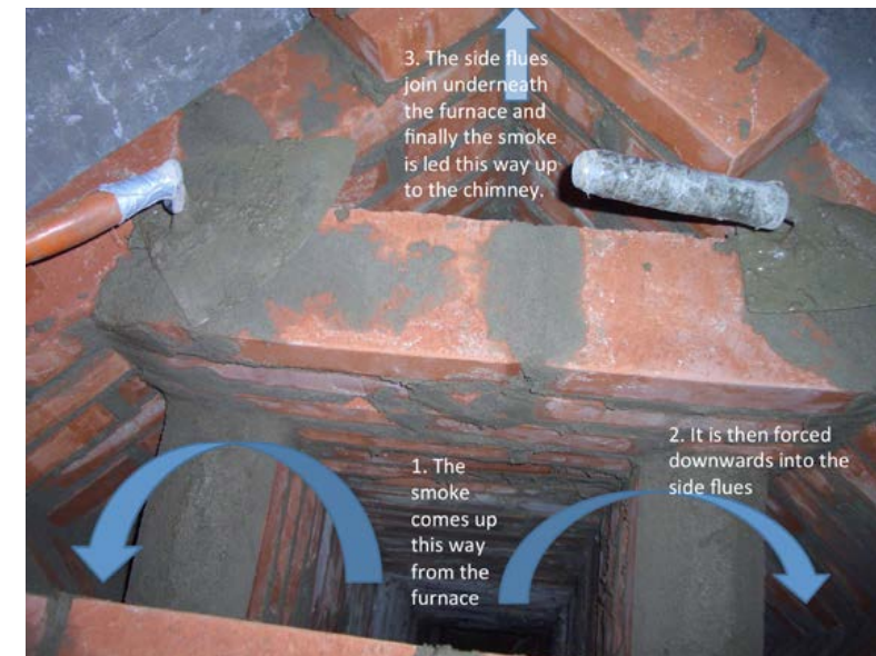
Figure 2.60. View down the flues at the level of tile row 4 (see also drawing). The next row of bricks will close the front flues.
