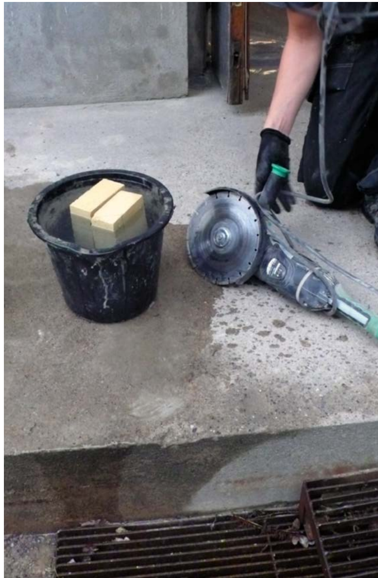
Figure 2.36. Before using the angle grinder the fireproof bricks are hydrated to avoid over-heating the blade.
