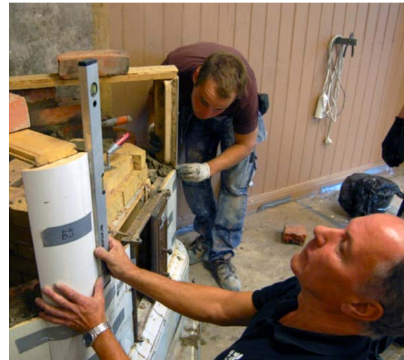
Figure 2.40. The corner tiles of tile row 9 are aligned with spirit levels. A small amount of mortar is placed beneath them before they are put in place. Master mason Krister Lindroos ( in the front ) assists with the difficult parts.
