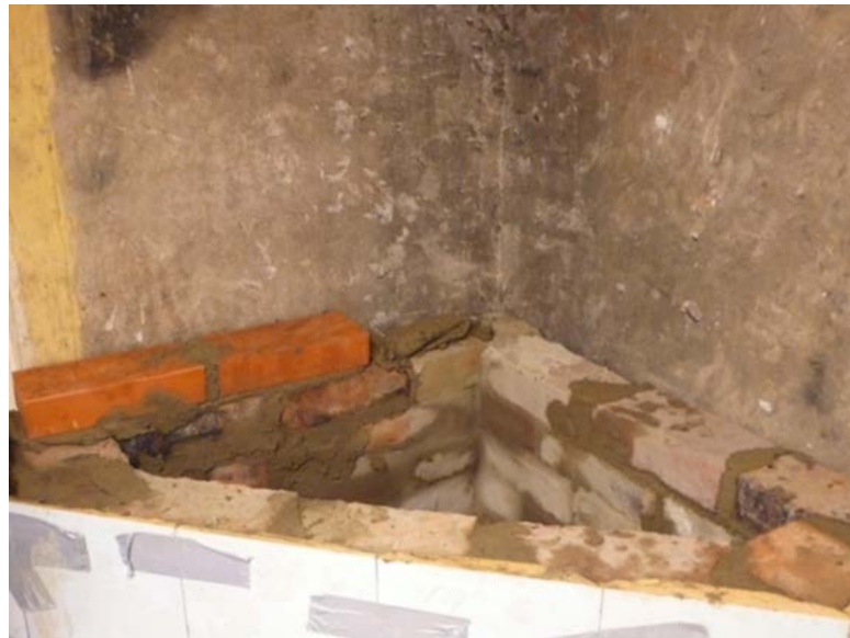
Figure 2.51. When we reached the top of tile row 7, we ran out of old bricks and started to use new PT-standard bricks.
