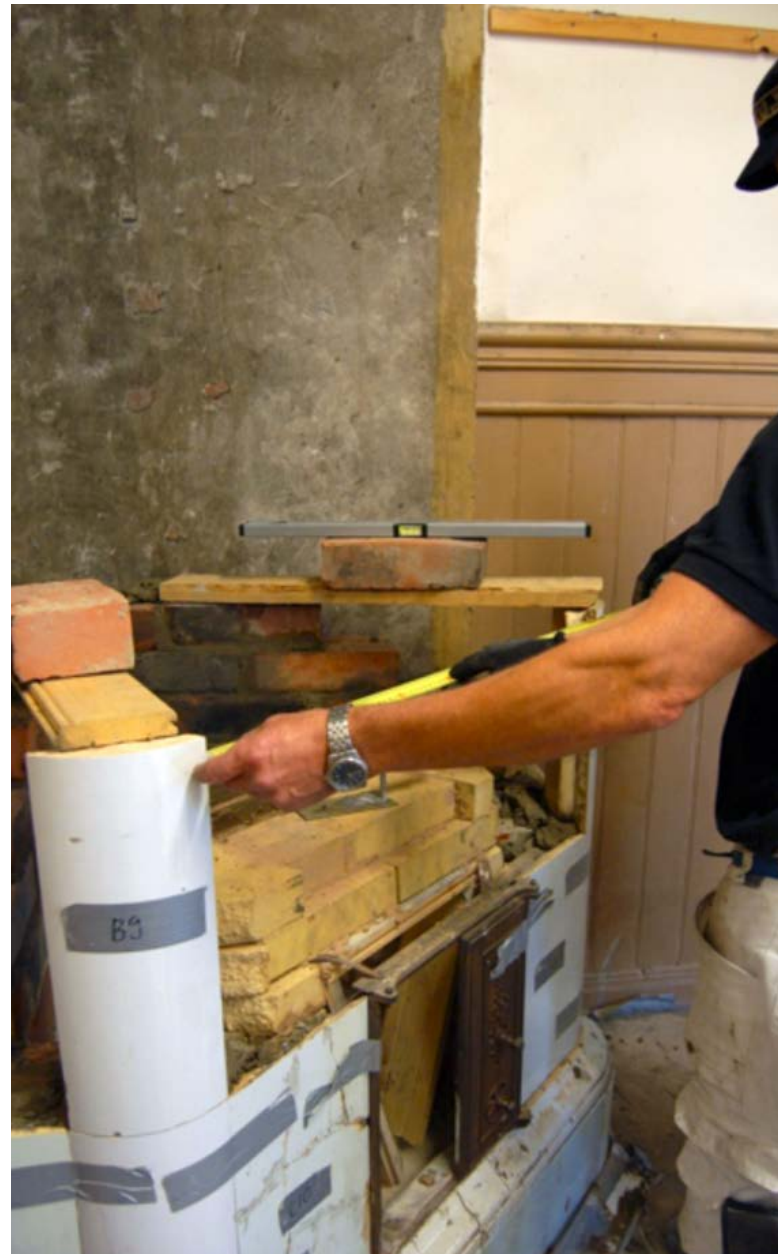
Figure 2.41. When both corner-tiles are in place the distance is double-checked to insure that the centre tiles will fit.
