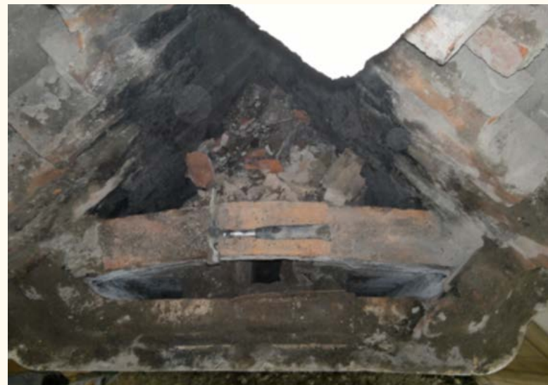
Figures 2.10 a, b. One row of bricks below the top of the fifth tile row: At last we can see the basic structure of the stove with its 5 flues. Above: measured drawing of the same.
