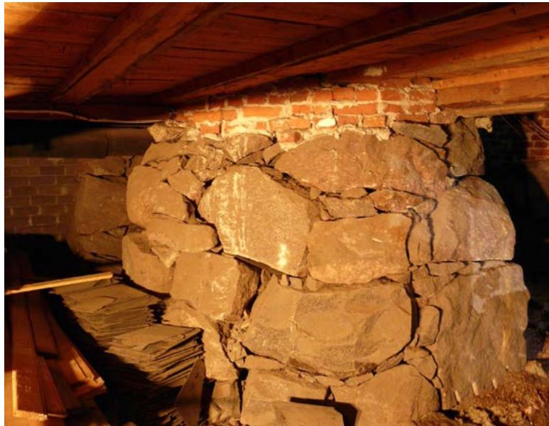
Figure 2.1. Every kind of stove or fireplace has to stand secure and immobile since movements in the masonry would lead to cracks and obvious fire hazard. This enormous dry laid foundation supports the stove whose dismantling and consequent rebuilding is described in the following. The stove itself weighs several tons.
