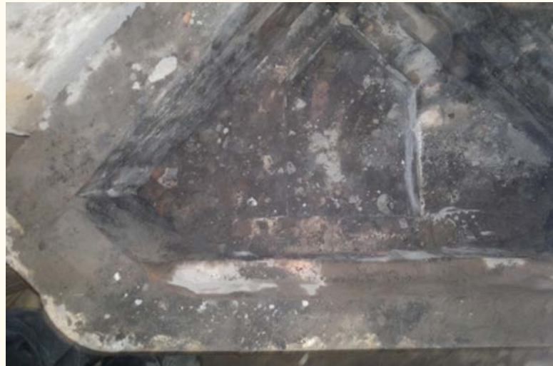
Figures 2.14 a, b. The ninth tile row is still in place but several rows of brick have been taken out from behind it. Here the floor of the furnace can be seen. This is where the dismantling was stopped because the bottom of the stove was intact and it was of course easier to start the rebuilding from a foundation that was of the correct size and shape. Above: measured drawing of the same.
