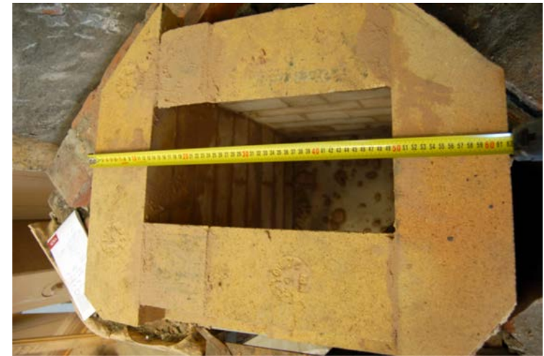
Figure 2.34. The middle flue is narrowed at the back and front of the furnace with a row of bricks that have been shaped with an angle grinder. This bottle neck will improve the draught in the flue.
