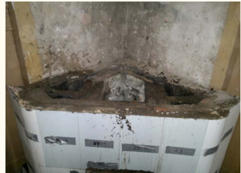
Figures 2.13 a, b. Top view of the ninth row of tiles. Here we can see the top of the furnace. Above: measured drawing of the same.
