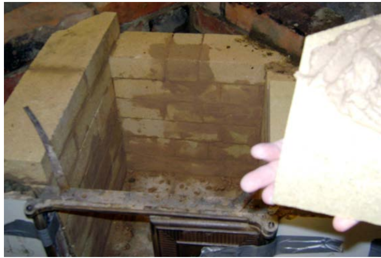
Figure 2.32. The fireproof bricks are built to the upper part of the cast iron frame of the shutters.
