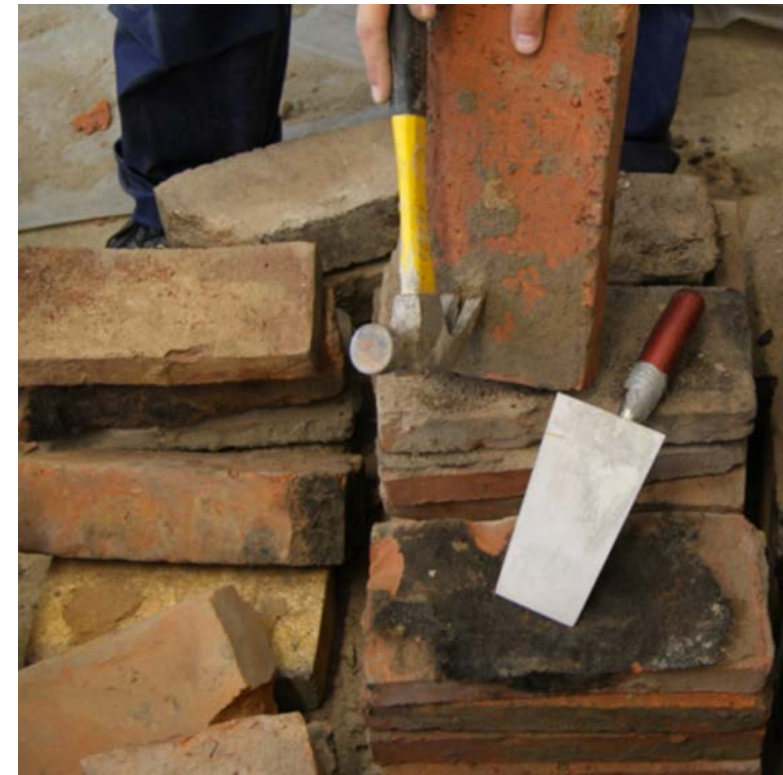
Figure 1.10. Cleaning the bricks is done by using a hammer and a trowel. Clay mortar comes off quite easily but the job is dusty and dirty.
