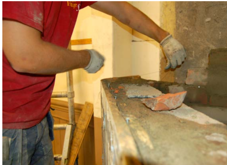
Figure 2.38. Nails are inserted into the existing holes in the flanges of each tile and tied together with a baling wire which is fastened in the joints of the rear brick course.
