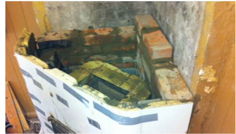
Figure 1.35. Interior of the stove at the end of day 1.
