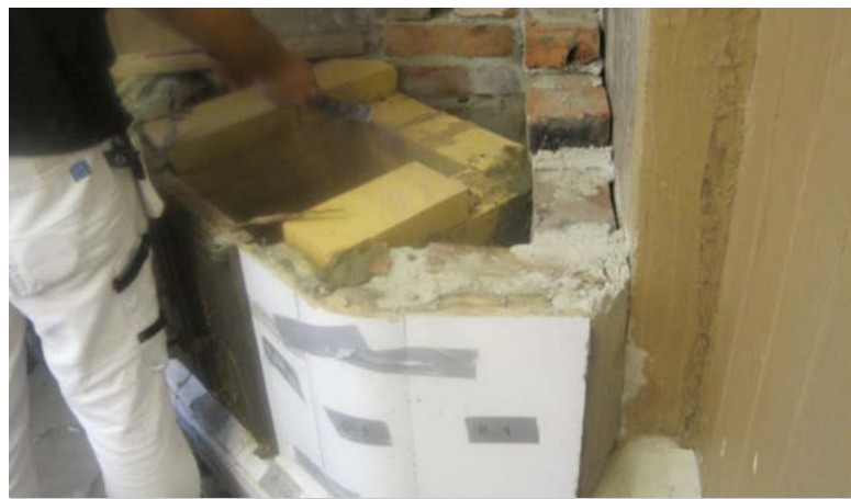
Figure 1.22. Laying the lower part of the furnace. Fireproof bricks and mortar were used. The masonry of the furnace should be bonded together with thin joints (1–2 mm) and separated from the rest of the masonry that has wider joints of clay mortar (13–15 mm).
