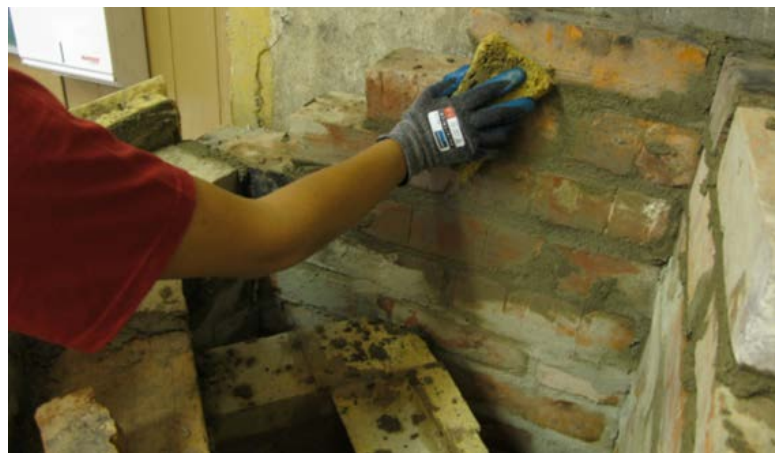
Figure 1.19. Washing off the clay mortar from the bricks in order to smoothen the walls of the flues.
