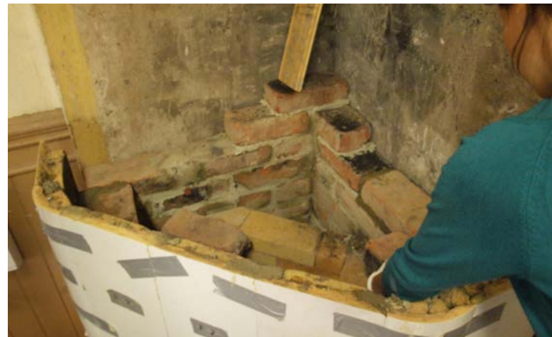
Figure 1.40. Five more rows of fire-proof bricks are layed up from the furnace. From then on the central flue is built using ordinary bricks and clay mortar.
