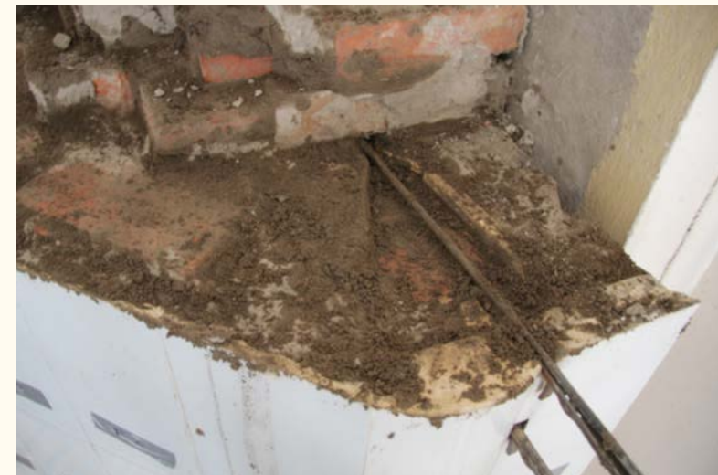
Figures 2.4 a,b. Two top rows of tiles have been removed and the top damper is now visible. Above: drawing of the same.
