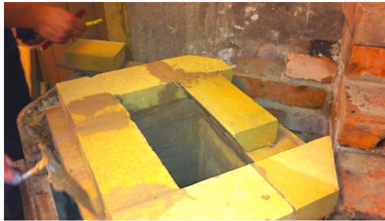
Figure 1.24. Installing the second row of sawn bricks.
