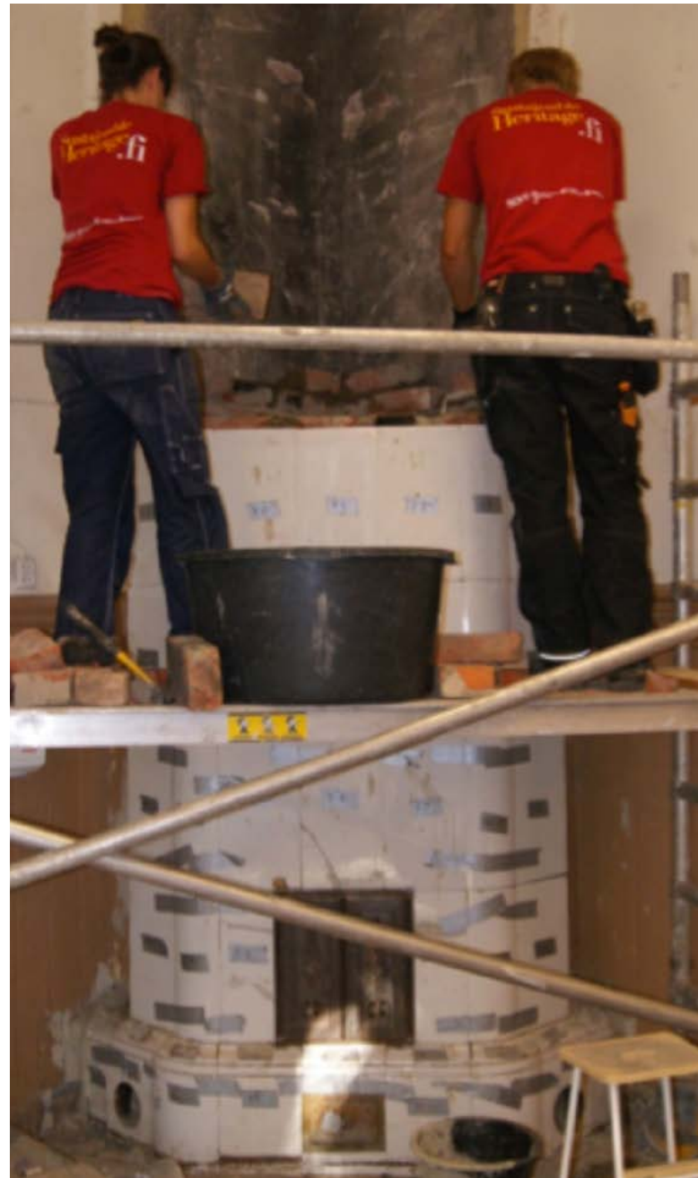
Figures 1.42–43. On day 4 two rows of tiles were installed.
