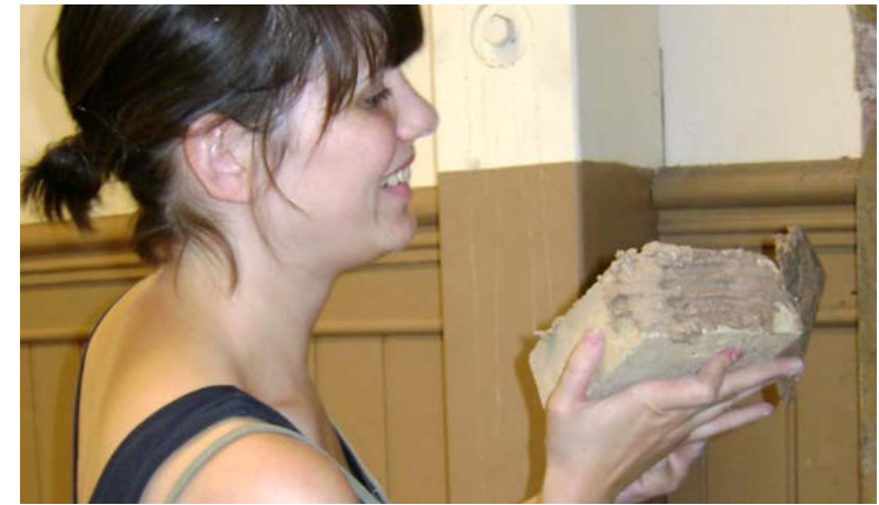
Figure 2.30. The fireproof mortar is applied directly on the fireproof bricks before they are put in place.
