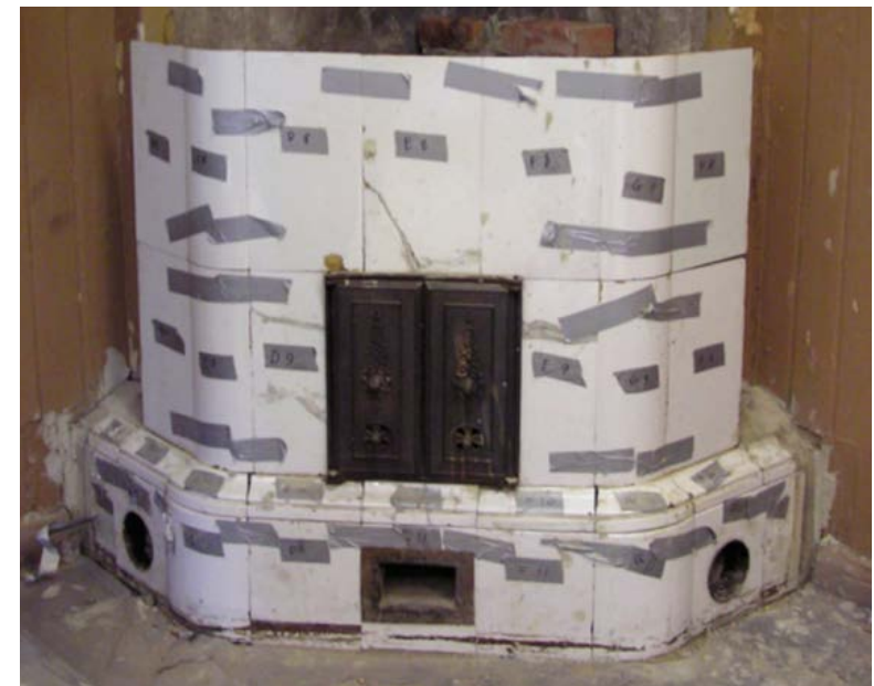
Figure 1.36. End of day 1. We had built our first row of tiles and the furnace behind it.
