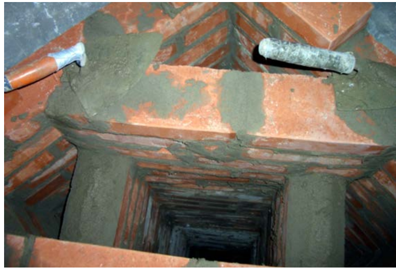
Figure 2.55. Looking down the system of flues just before the top was closed with solid brickwork.
