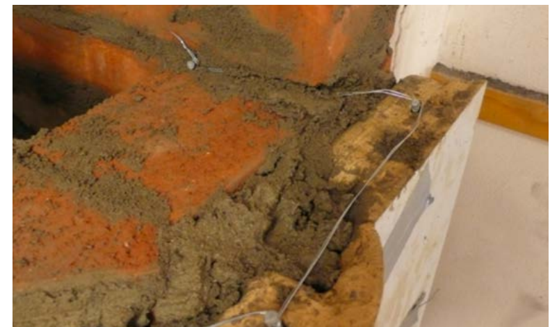
Figure 2.54. The wire is secured by a nail in the mortar joint of the side wall of the stove.
