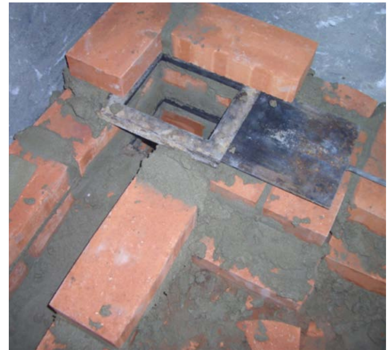
Figure 2.57. Tile row 3: the two dampers can be seen at the start of the chimney. To the left we have built the air duct for summer ventilation. (See also drawings.)
