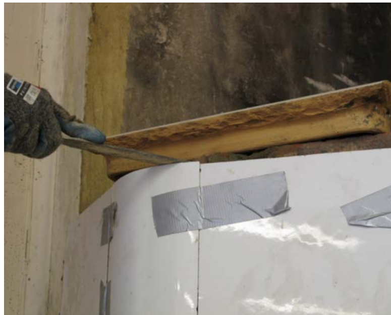
Figure 1.30. Correcting the size of the tiles can be done either by filing or using an electric saw.
