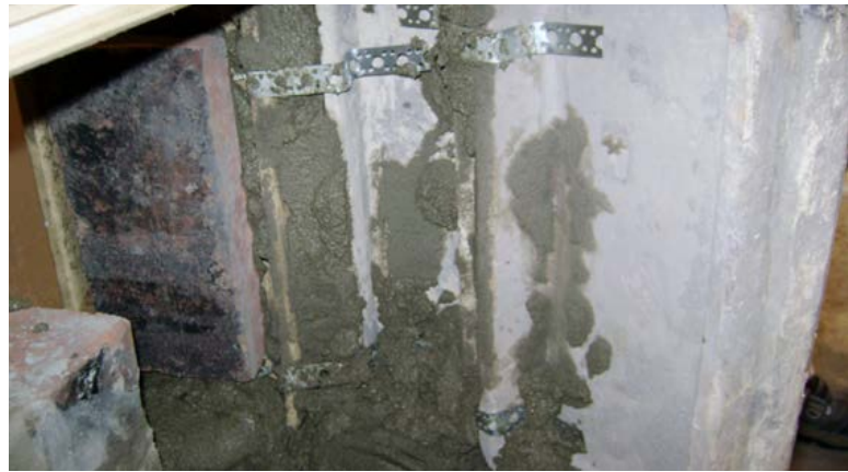
Figure 2.26. The cavity behind each tile is filled with thin bricks and clay mortar.
