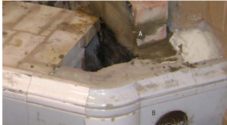
Figure 2.22. (A) The bricks are laid with clay mortar and with a 2 cm wide gap between the fire wall and the backside of the stove. (B) At the bottom of each side flue there is an opening with a metal cap. When the chimney (in the back corner of the stove) is swept the soot can be removed through these horizontal flues. The side cannels also join underneath the furnace floor and lead to the chimney in the back.
