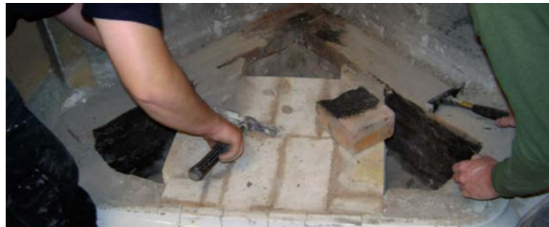
Figure 2.21. This is where we started the rebuilding of the stove. The bottom two rows of tiles were already in place (they were intact and therefore not dismantled). Before laying new bricks the base had to be cleaned and the old mortar removed.
