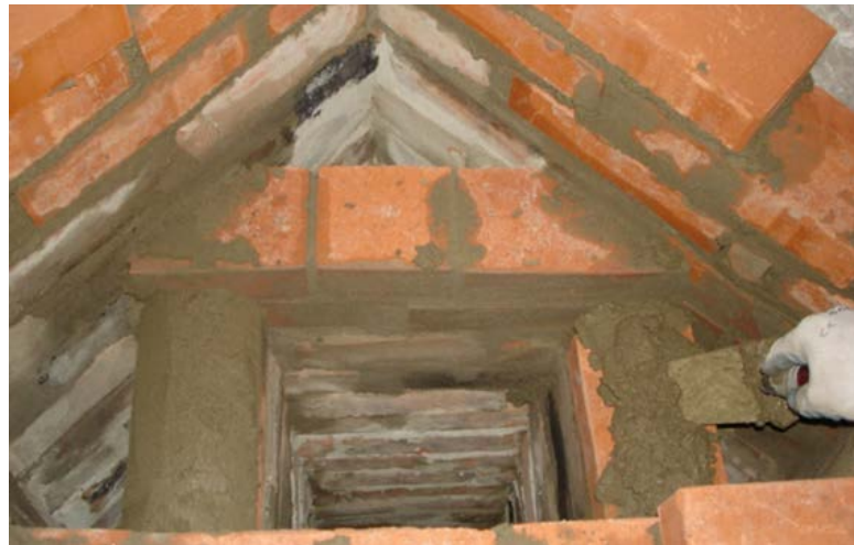
Figure 1.44. Day 5. Finishing the central flue just before installation of the last row of flat tiles. The tops of the side walls of the central flue are rounded to direct the air-flow to the flue pipes.
