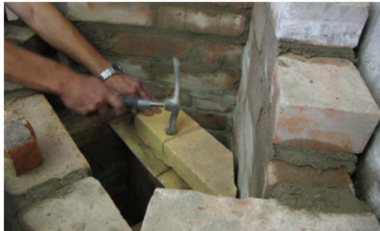
Figure 1.18. A hammer is used to adjust the bricks and tighten the joints.
