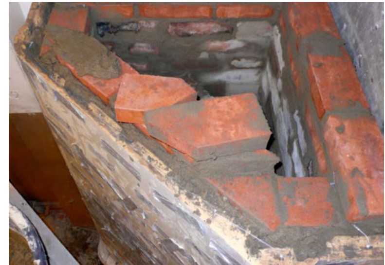
Figure 2.53. One and a half courses of the new bricks were laid. Before continuing the baling wire was attached as described before.
