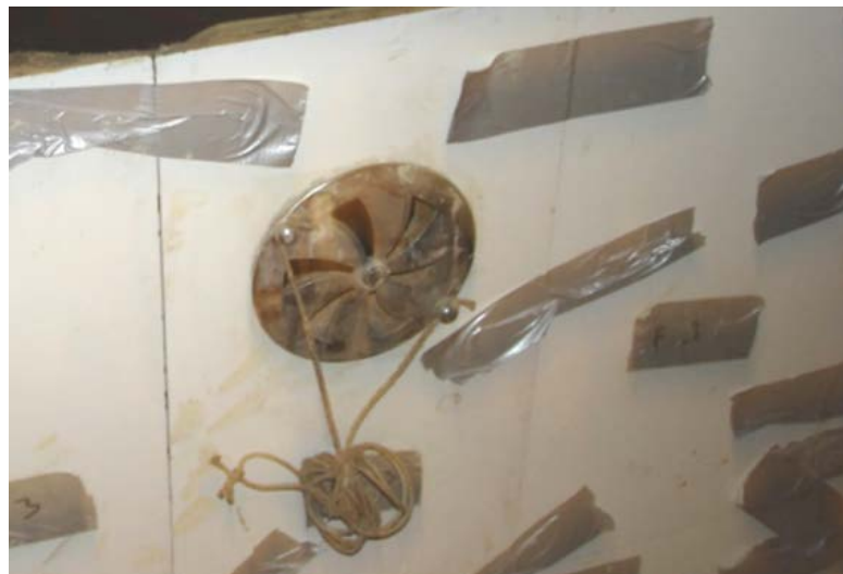
Figure 1.45. Rosette air vent in the last row of tiles before installing cornice.
