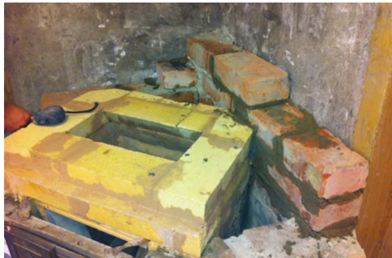
Figure 1.25. Continuing the laying of bricks at the rear. The gap between the fire wall and the rear masonry works as an insulator which keeps the warmth from transferring into the walls. It also allows the bricks to expand without breaking the stove.
