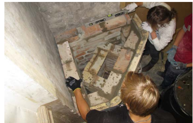
Figure 1.17. A spirit level should be used to level the bricks and help make the structure straight and secure.
