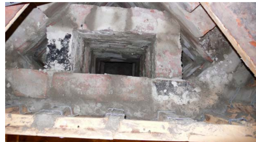
Figure 2.50. A view down the inside of the stove from the level of tile row 6.
