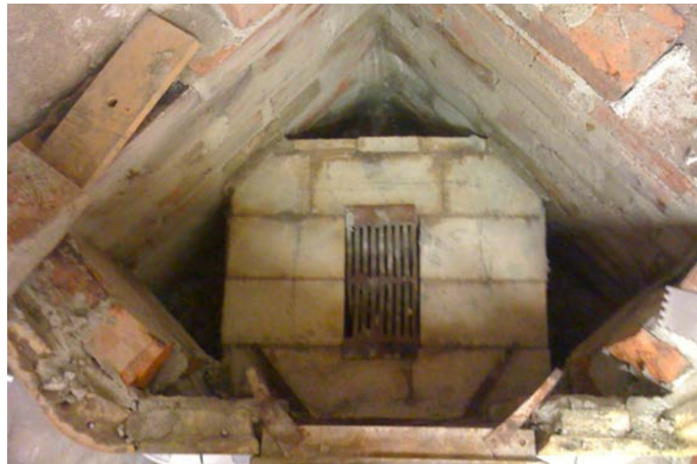
Figure 1.21. The interior of the stove showing the floor of the furnace.
