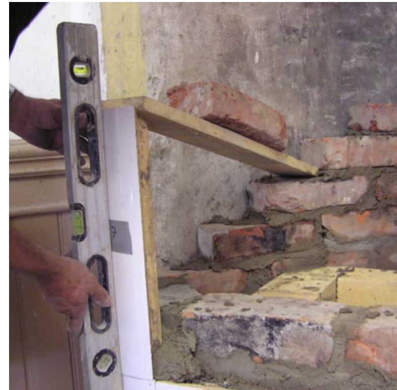
Figure 1.28. Corner tiles are the first to be installed. Therefore it is important to compare the distance between them with the width of the middle tiles. To keep the first tile in the right position and angle, it needs to be pressed downwards. A board with a weight is used. This is why the rear masonry needs to be built before the tiles are placed.
