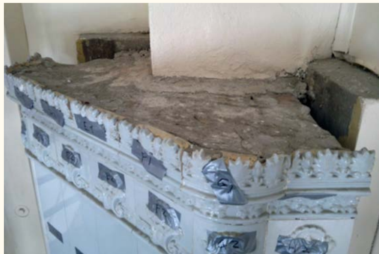
Figures 2.3 a, b. View of the top of the tiled stove before we began dismantling it. Above: a measured drawing of the same. Note the masonry fire walls that separate the stove from surrounding log constructions.
