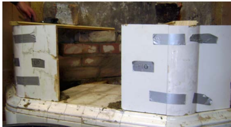
Figure 2.27. Our first row of tiles, marked number 10, is in place. Tape is used to hold the tiles until the mortar has set.
