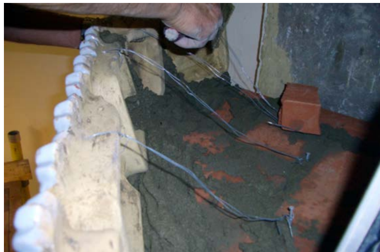
Figure 2.59. The masonry work for the stove is finished when these wires are finally covered with bricks and mortar.
