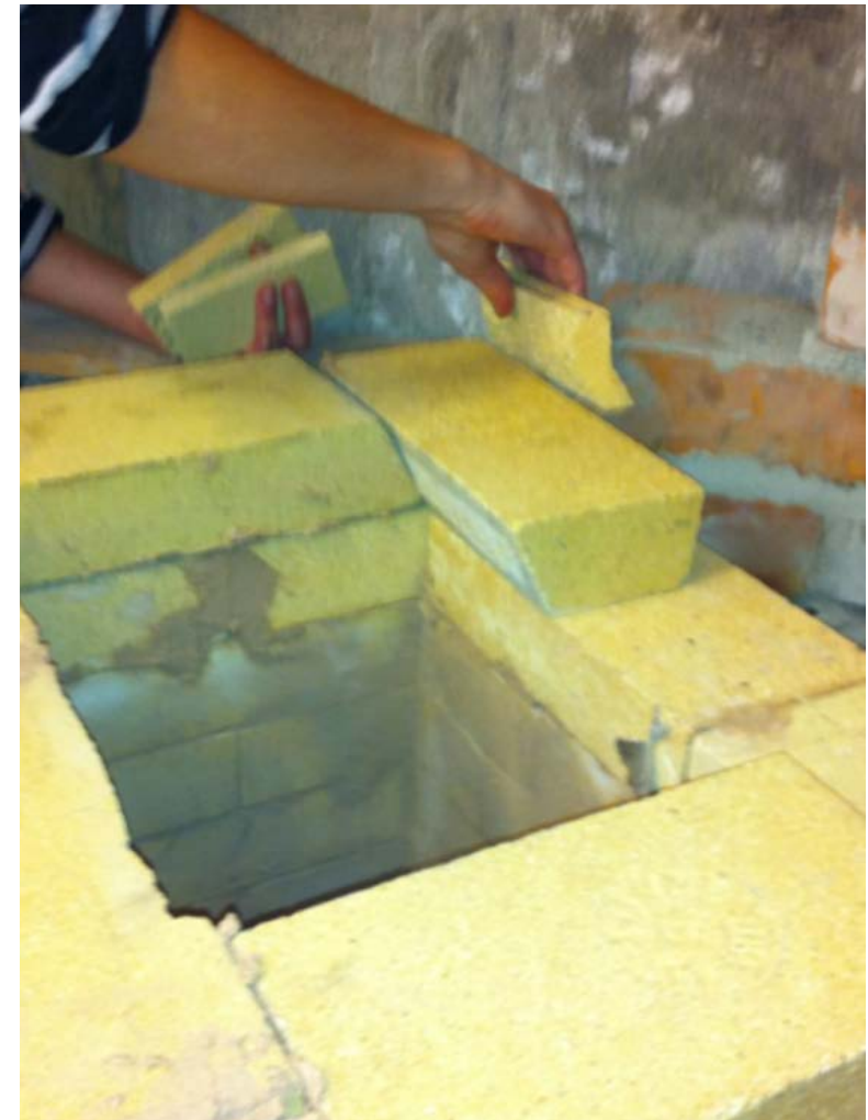
Figure 1.23. The rear masonry was laid to the height of half of the next tiles to be used as a support for the tiles.
