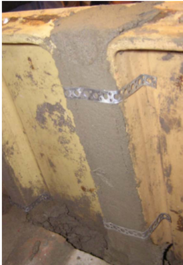
Figure 1.32–33. When the tiles are in place, the gap between them is filled with clay–mortar. Then two clamps made of perforated metal strap are bent to hold them together. The cavity on the backside of the tiles is then filled with mortar and thin bricks. Inside this a wall of bricks is built to finally stabilize the front.
