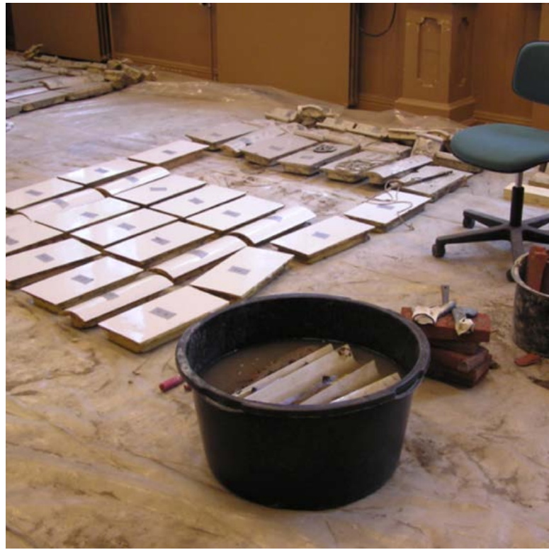
Figure 1.11. The tiles were soaked in water to soften the mortar. Three rows of the tiles on the floor have been cleaned and the lower rows of tiles are already assembled on the stove.
