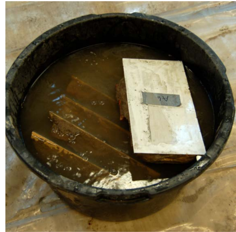
Figure 2.17. The rebuilding of the stove started with removing the mortar from the tiles and the thin bricks in the cavity on the back of each tile. The tiles are sunken in water for about half an hour in order to soften the old mortar before they are washed and cleaned. This is why it is important to use clay mortar: cement would not dissolve in water and the tiles would crack if they were cleaned with force.
