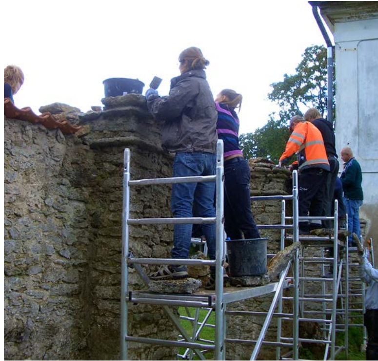
Figure 2.9. Estonian students working on gatepost C in the front; Finnish students in the middle, studying post B, and Swedish students busy with post A in the background.
