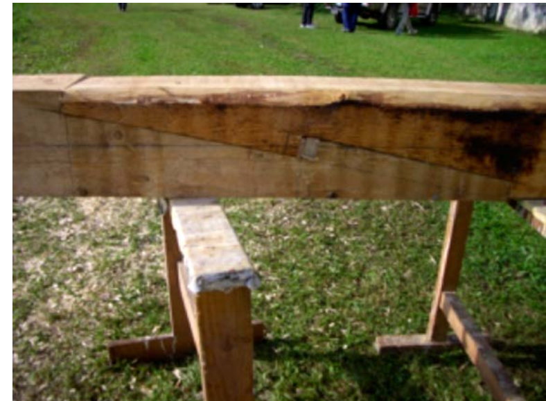
Figure 3.30. The finished joint.
