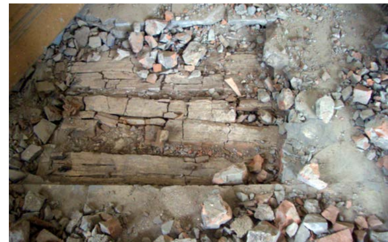
Figure 3.2. Seidla Manor. Floor boards are cracked by fungi. The topmost layer of bricks and plaster has not allowed rising damp to evaporate from the underlying wooden construction.
