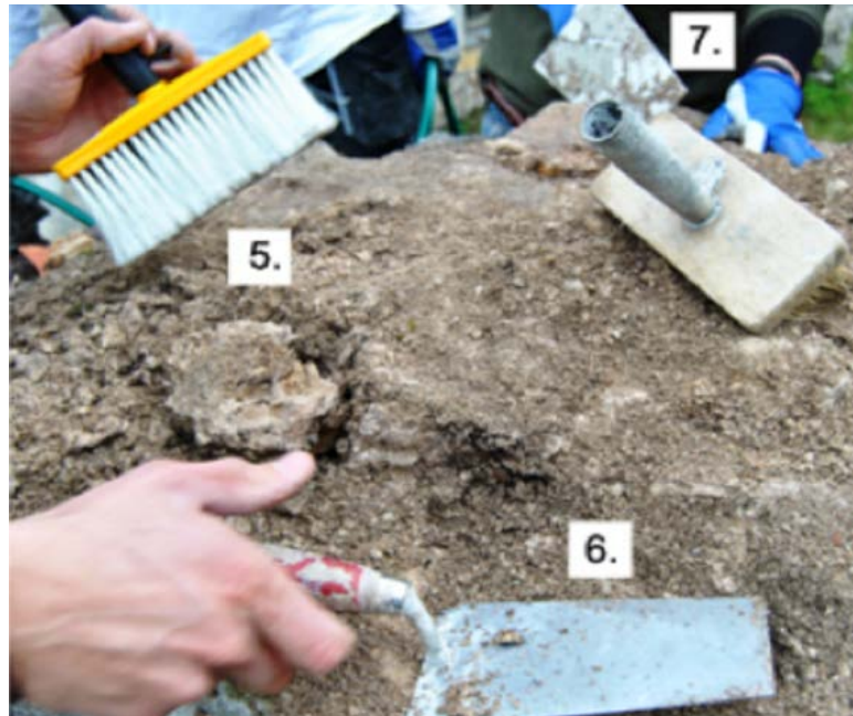
Figure 2.11. More tools: brushes (5)—used to wipe off sand and also to even out mortar on the sides of the posts; trowels (6)—used to apply the mortar onto the wall; waterproof gloves (7)—used when handling the mortar to prevent direct contact with lime; tape measures used for documentation.
