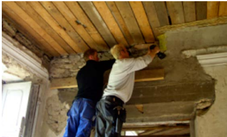
Figure 3.44. Reconstructing a cornice in one of the badly damaged rooms on the upper level.
