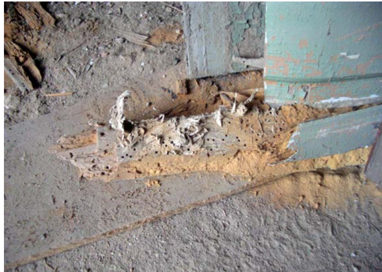
Figure 3.3. Seidla Manor. Top left: brown rot; center: white rot and destruction by wood boring insects.
