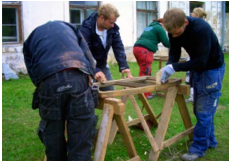
Figure 3.35. Sandpapering was quite easy as there was only one coat of paint to be removed and the wood was mostly in good condition.
