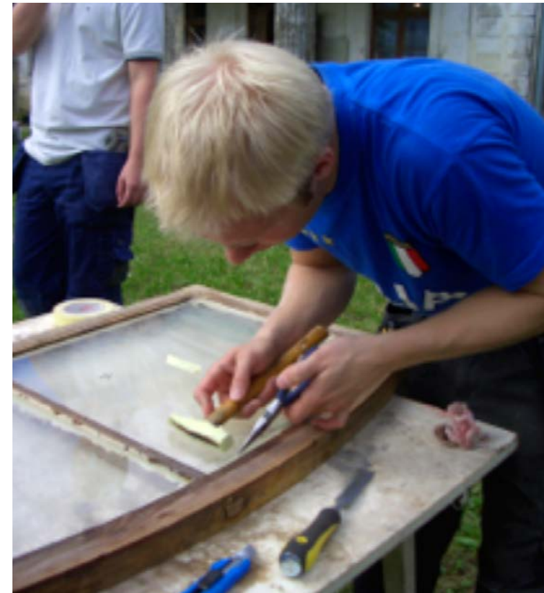
Figure 3.36. Nails are being inserted. The small hammer is wrapped in masking tape to avoid scratches on the glass.
