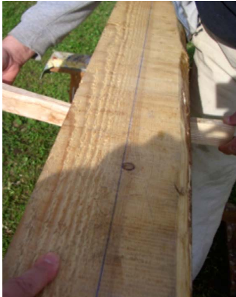
Figure 3.28. Finally we put the pieces together and secure the lock made of two wedges.
