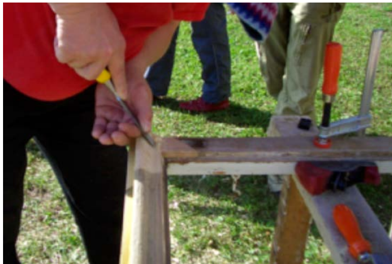
Figure 3.38. The new patch of the weather moulding is being shaped to match the old parts.
