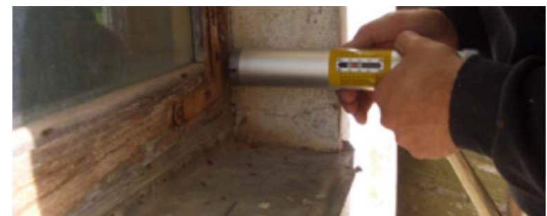
Figures 3.15–16. The Pilodyn was tested on timber with various degrees of decay.
