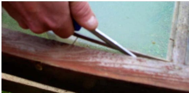
Figure 3.33. A glazing bead is being removed.
