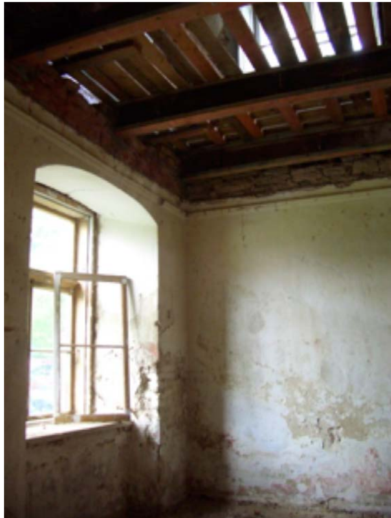
Figure 3.39. In some of the rooms at Seidla Manor there was neither ceiling nor cornice. Everything needs to be rebuilt.
