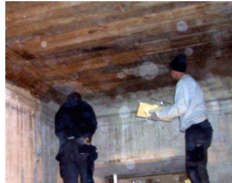
Figure 3.46. We were given a chance to try the traditional method of plastering the reconstructed cornice. This job is definitely something for experts!
