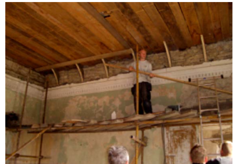
Figure 3.43. In the upper hall: new consoles are in place and planks are being attached to these. We finished the woodwork for the cornice along one wall.
