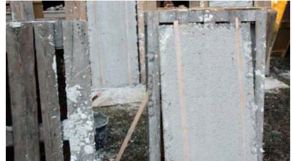
Figure 14. Creating an even surface by using two strips of wood as guide.
