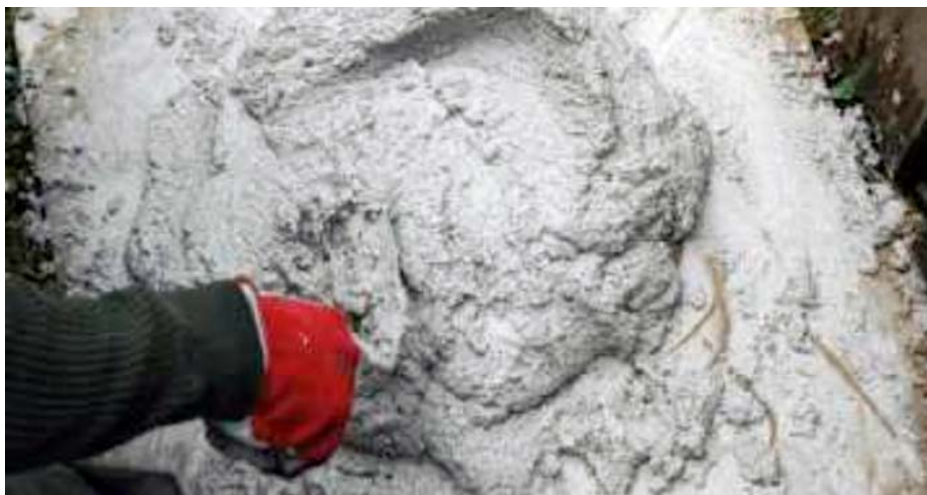
Figure 10. Mixing hot lime by hand.
