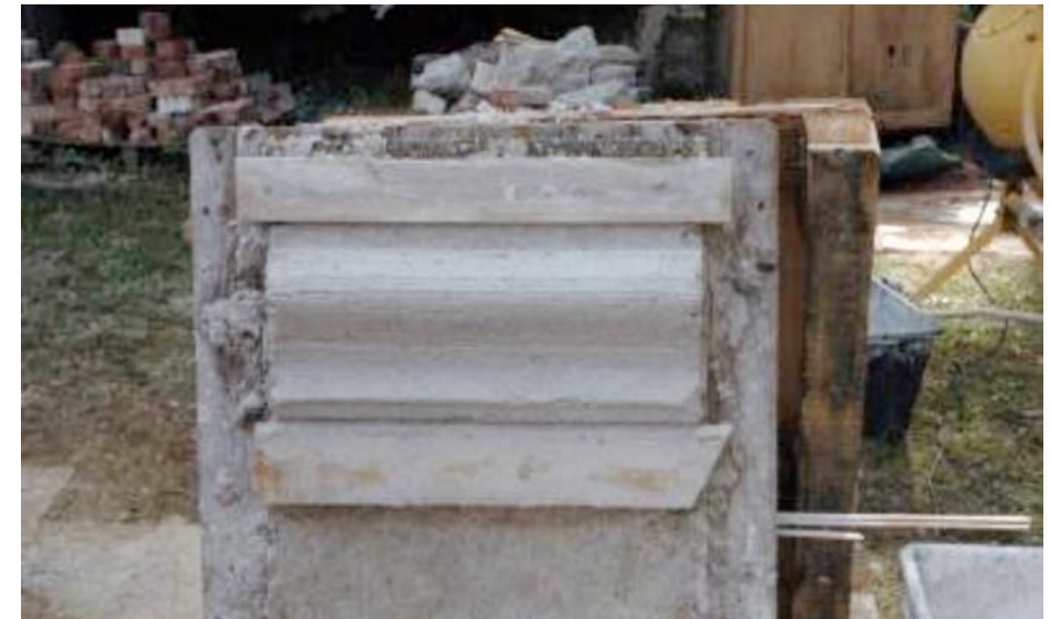
Figure 15. Moulding the surface by using a stencil.
