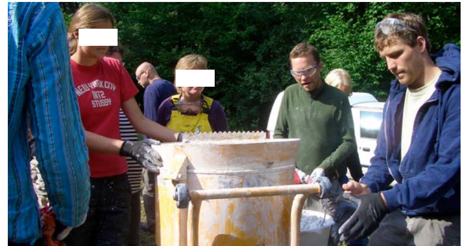
Figure 12. Making bigger quantities of lime render by using a roller pan mortar mill.
