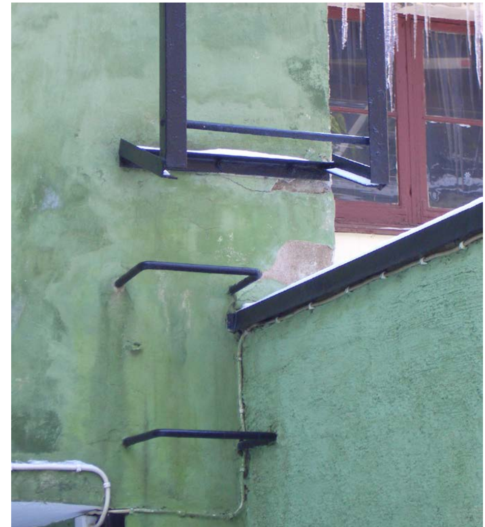
Figure 4. Multiple problems on both rendering and lime wash caused by bad detailing, rain and frost.
