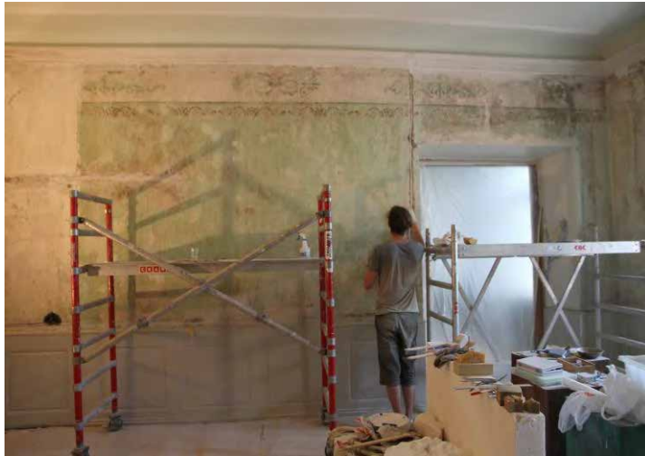
Work with filling holes with plaster continued. Photo: Rebecca Vemdal
