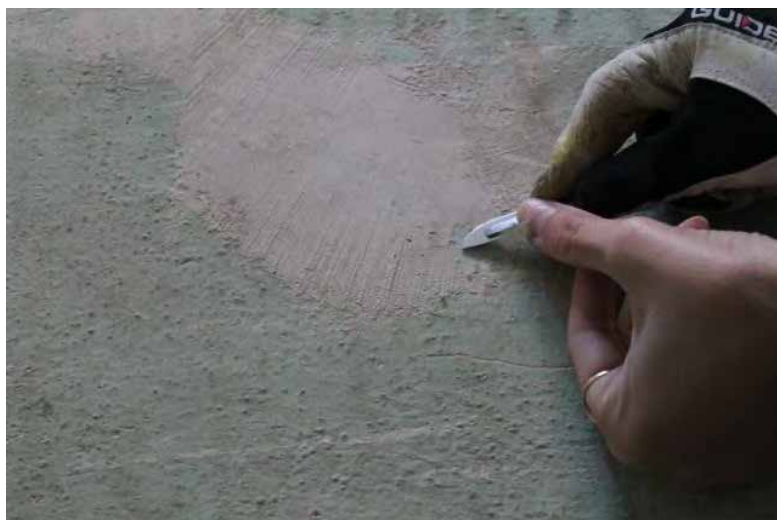
Photos depicting the process of revealing the green paint layer.
