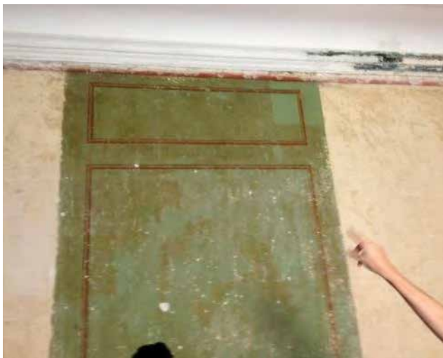
Wallpaper glue residues test cleaning. Photo: Anna Holmberg
