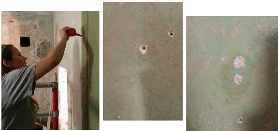
Air pumping the dirt away from the holes. Pictures of holes on the W-wall painting and holes filled up with plaster. Photos: Josefine Israelsson
