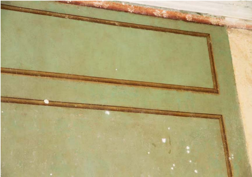
Dried plastered holes ready for retouching with paint. Photo: Vikoria Arvidsson
