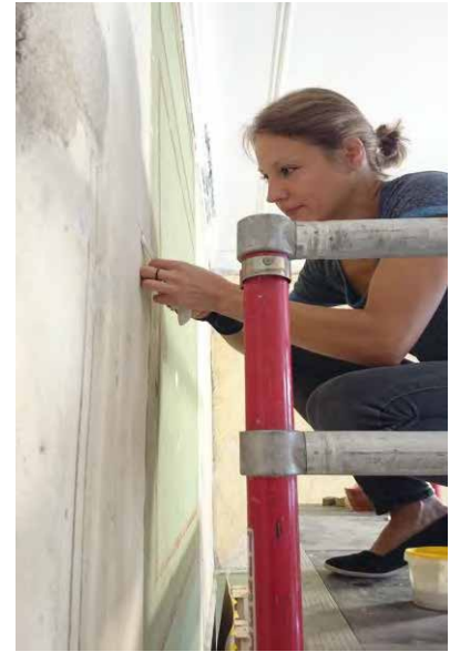
Filling of small holes in room N16 Photo: Rebecca Vemdal
