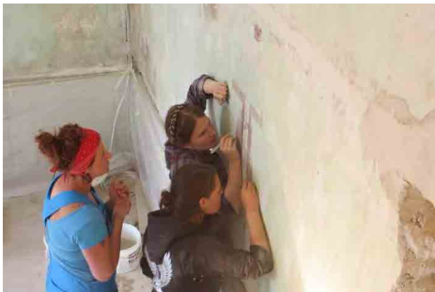
Exposing sample areas of the first wall painting. Photos: Taavi Tiidor
