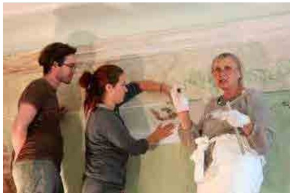
Heli is using a sachet with pigment to attach it to the wall using the pinned through stencil. Photo: Viktor Källgren
